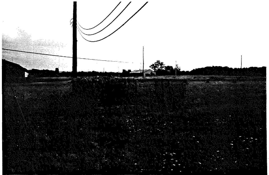
Photo 9: SEAD-4, 9/13/90. View of the Munitions Washout Facility Leach Field, facing south.
