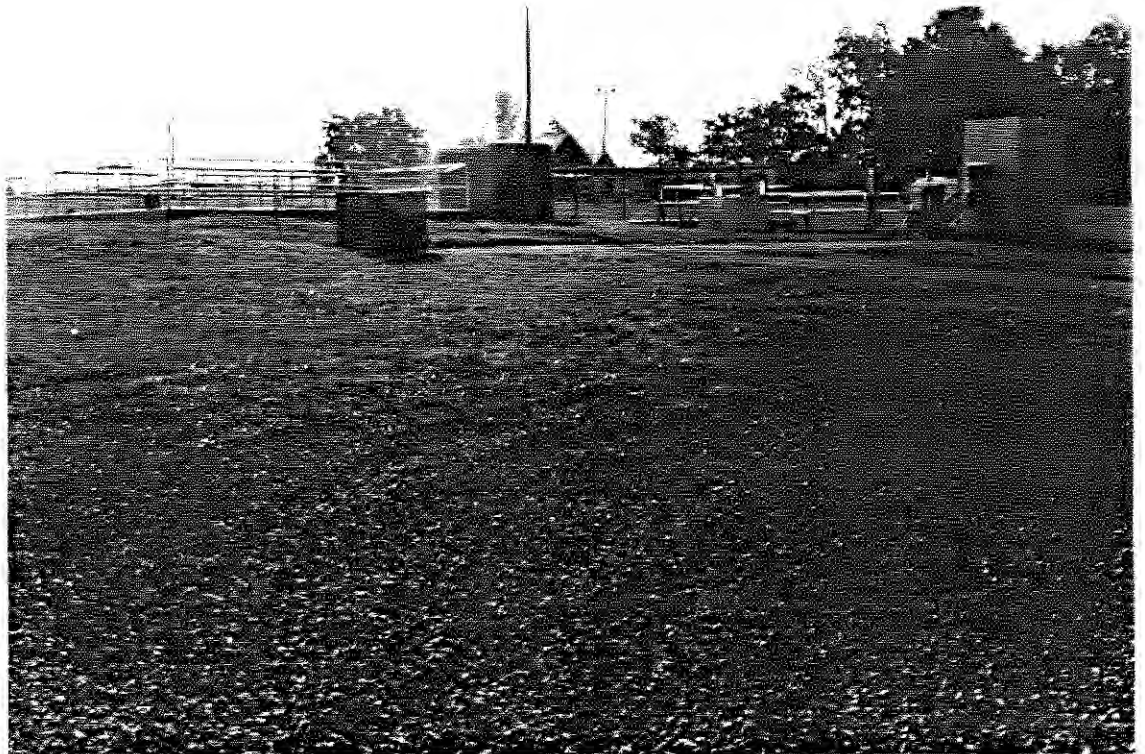
Photo 58: SEAD-21, 9/13/90. View of Primary Treatment - Sewage Treatment Plant No.715, facing east.
