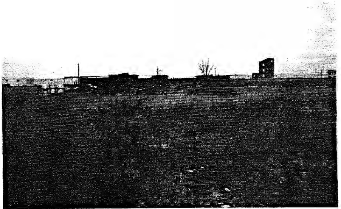
Photo 159: SEAD-64, 11/27/90. View of Location A of Garbage Disposal Areas, Debris Landfill south of Storage Pad, facing north.
