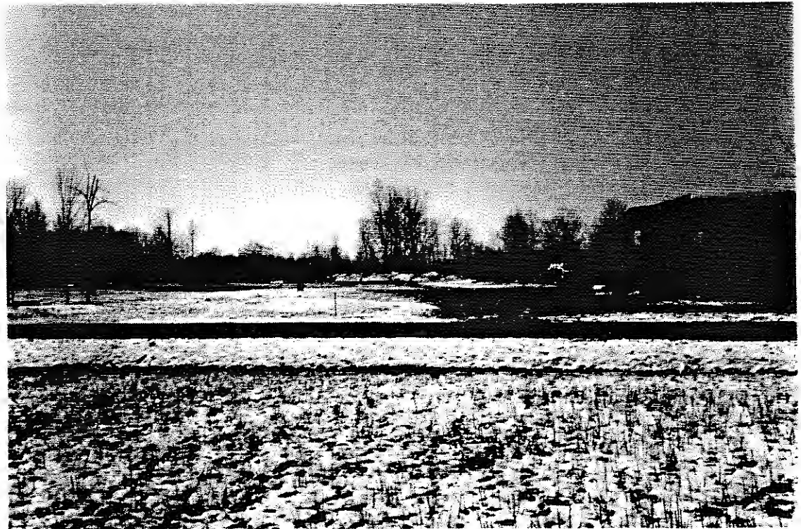
Photo 187: SEAD-70, 4-5-94. View of the western portion of the filled area and a portion of Building 2110, facing south.
