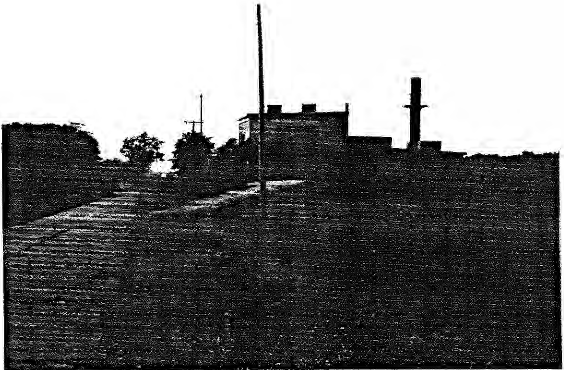
Photo 41: SEAD-15, 9/10/90. View of the Abandoned Solid Waste Incinerator - Building 2207, facing northwest.
