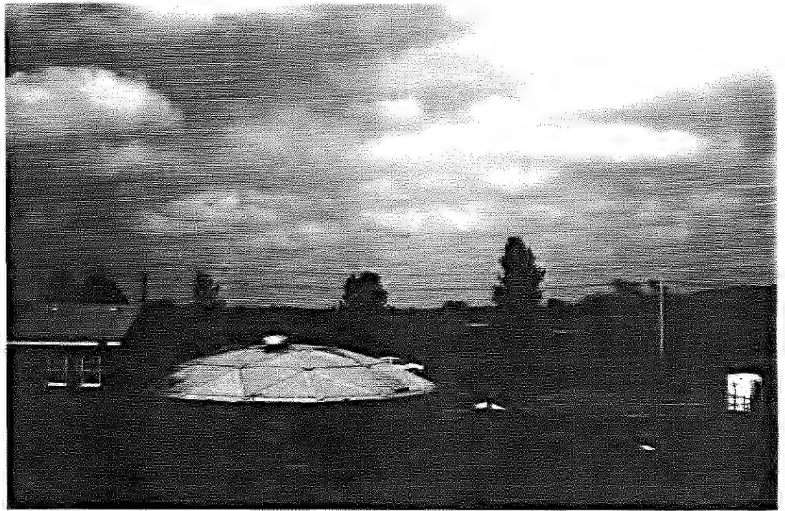
Photo 53: SEAD-20, 9/11/90. View of the Sewage Treatment Plant No.4, facing north.
