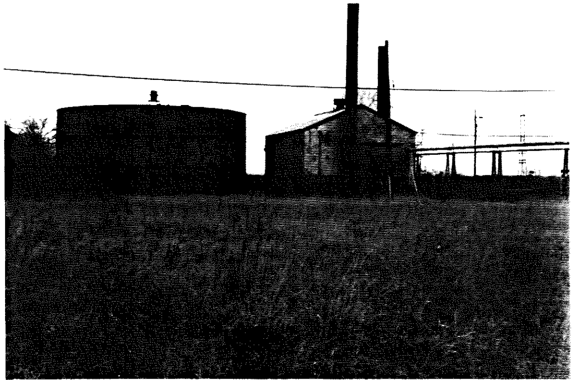
Photo 8: SEAD-4, 11/29/90. View of the Munitions Washout Facility Leach Field, facing northeast.
