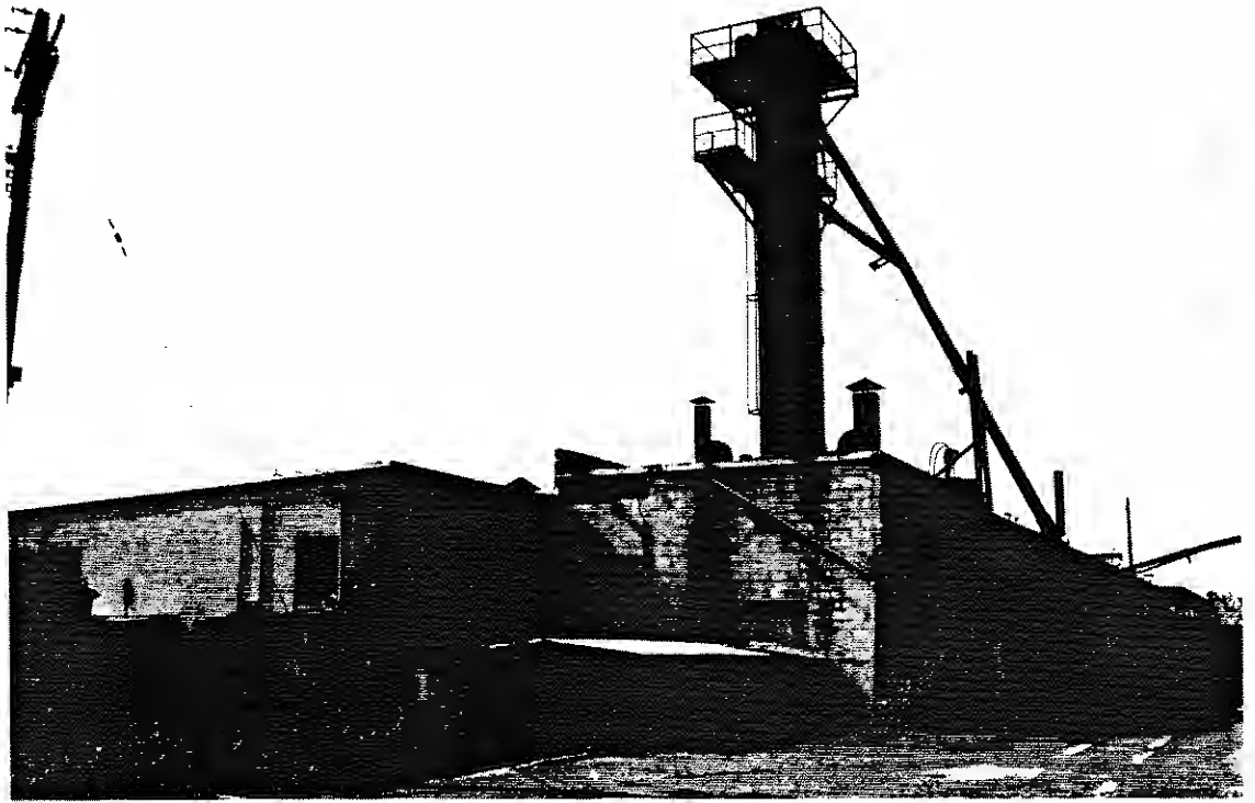
Photo 44: SEAD-16, 9/13/90. View of the Abandoned Deactivation Furnace - Building S-311, facing northwest.
