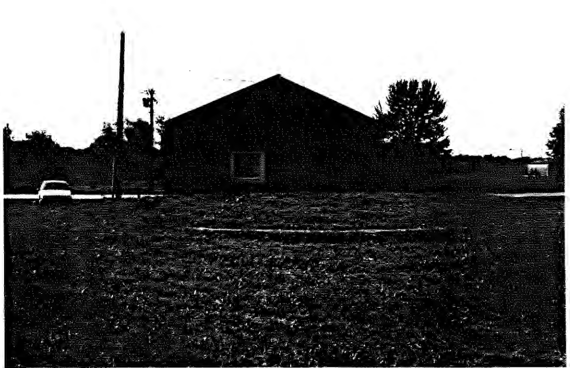
Photo 63: SEAD-22, 9/13/90. View of the trickling filter, Sewage Treatment Plant No.314, facing south.
