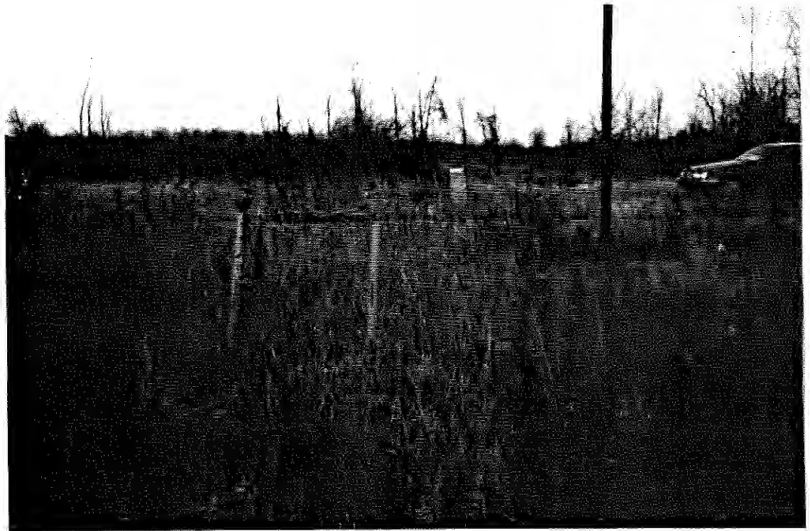
Photo 113: SEAD-44, 11/29/90. View of Location B of the Quality Assurance Test Laboratory, facing east.
