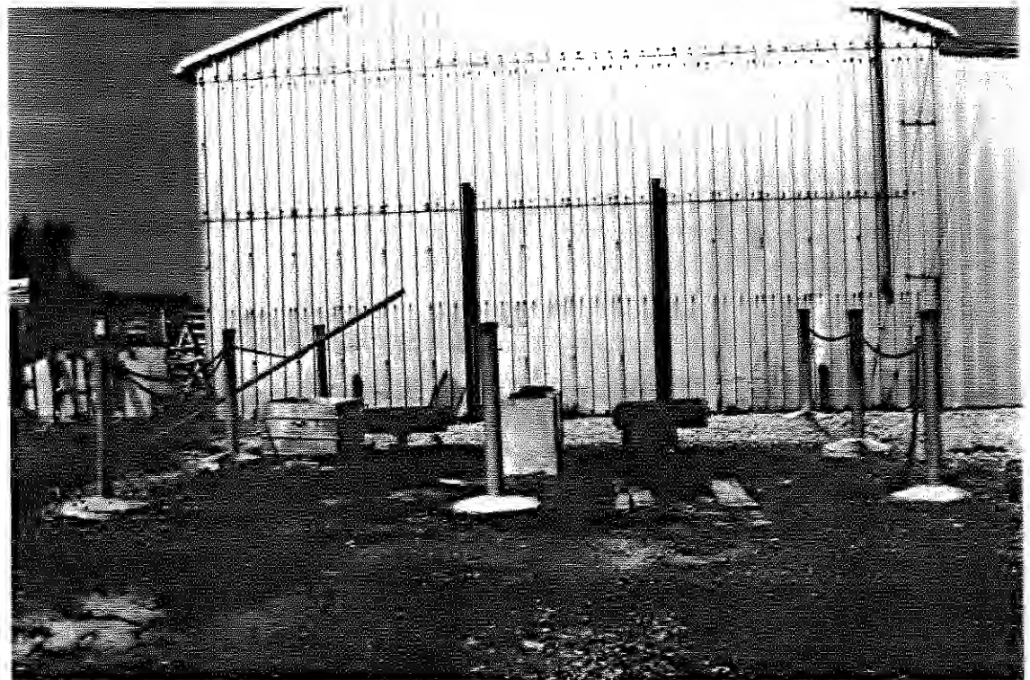
Photo 84: SEAD-28, 9/12/90. View of the location of two Underground Waste Oil Tanks - Building 360, facing northeast.
