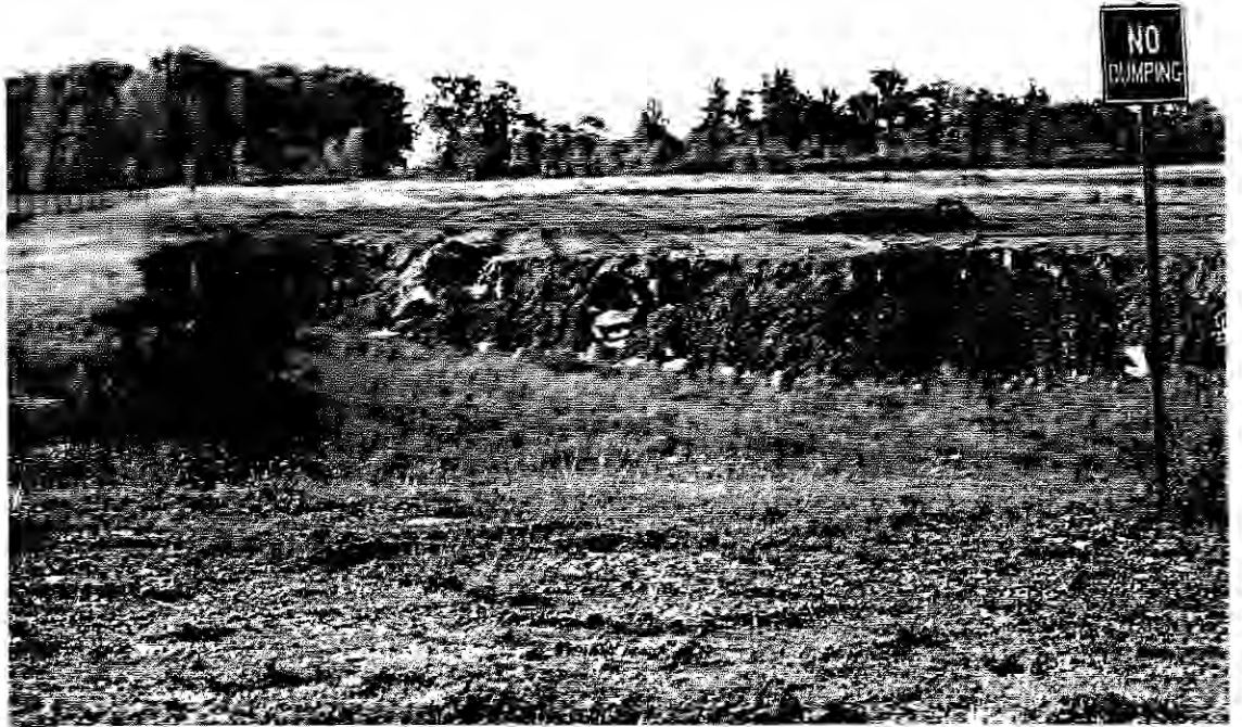
Photo 20: SEAD-7, 9/13/90. View of the Shale Pit, facing southwest.
