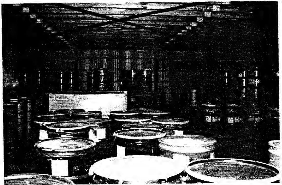
Photo 3: SEAD-1, 11/27/90. Interior of the Hazardous Waste Container Storage Facility - Building 307, facing northeast.
