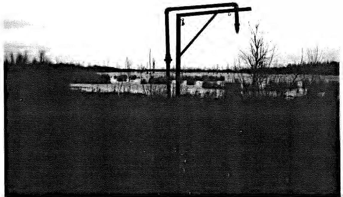
Photo 36: SEAD-13, 11/27/90. View of the aboveground piping observed on the southwest side of the Duck Ponds, facing north. The piping may be the deluge shower referred to in the 1960 IRFNA Disposal Report. Similar piping was observed on the southeast side of the Duck Ponds.
