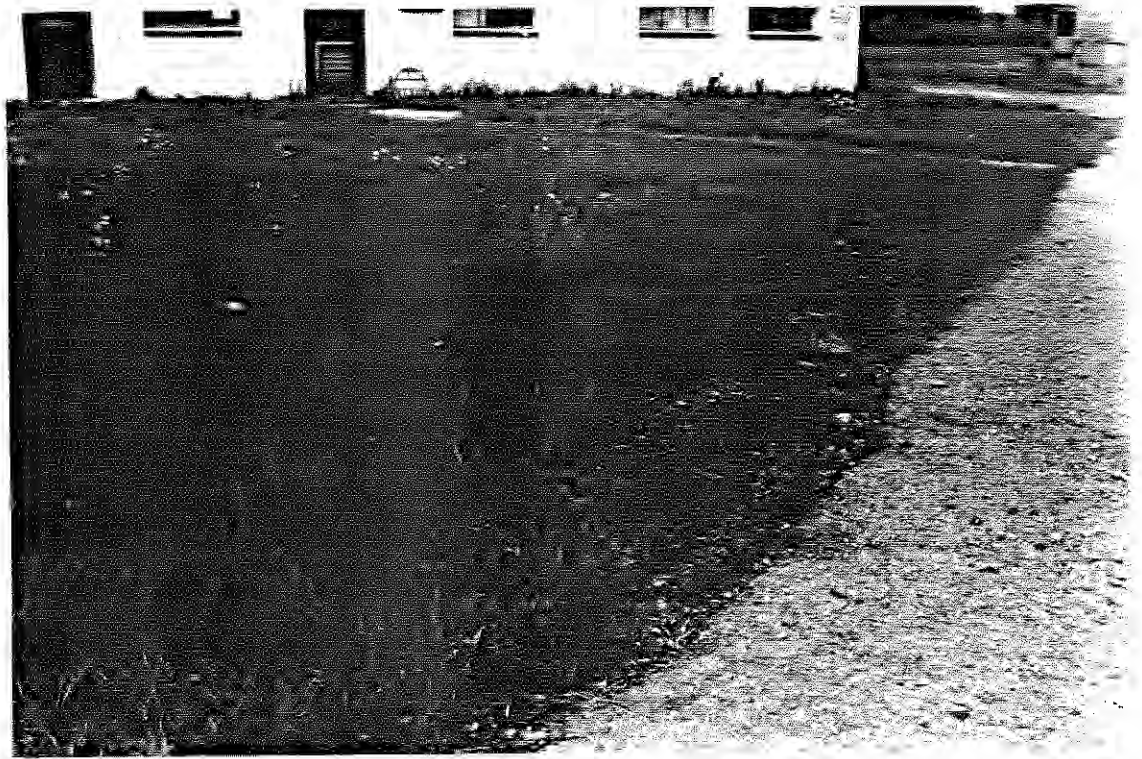
Photo 131: SEAD-56, 9/12/90. Stressed vegetation located close to the Herbicide and Pesticide Storage Area - Building 606, facing north.
