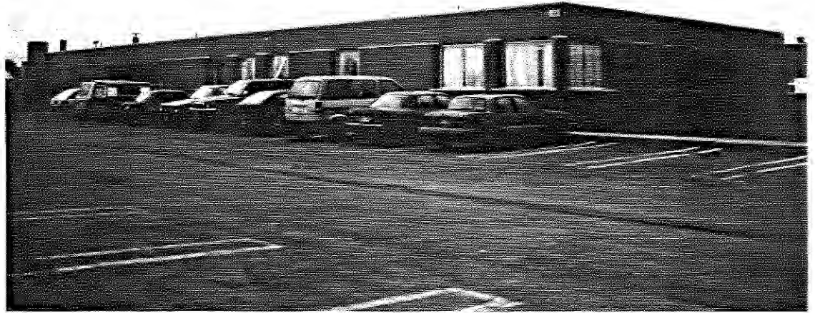
Photo 106: SEAD-42, 9/14/90. View of Building 106, where the Preventive Medicine Laboratory is located, facing southeast.
