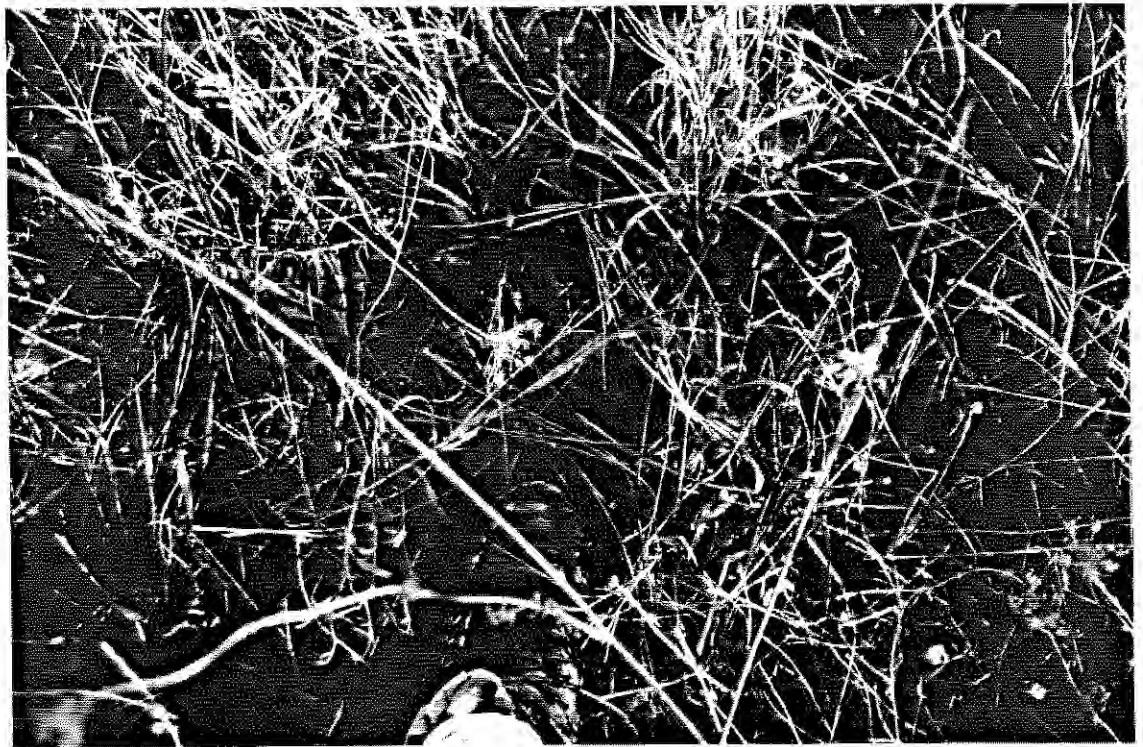
Photo 169: SEAD-65, 11/29/90. View of concrete foundation, Location B, Acid Storage Facility.
