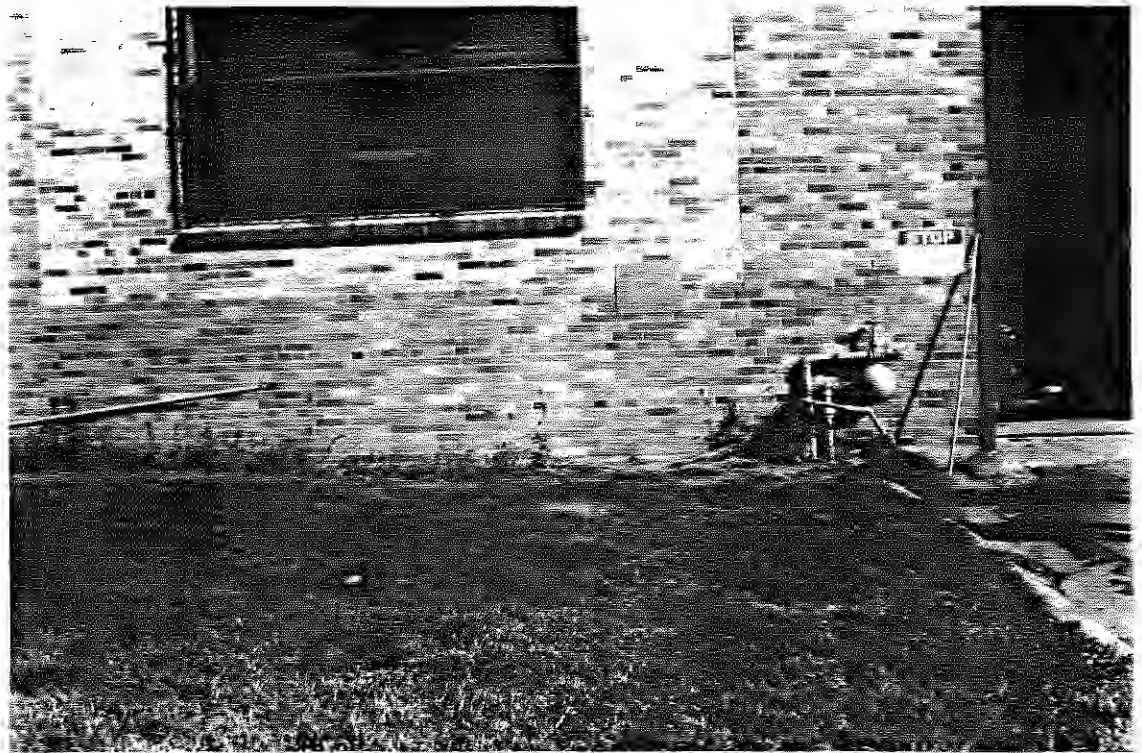
Photo 88: SEAD-30, 9/13/90. View of the location of the Underground Waste Oil Tank - Building 118, facing north.
