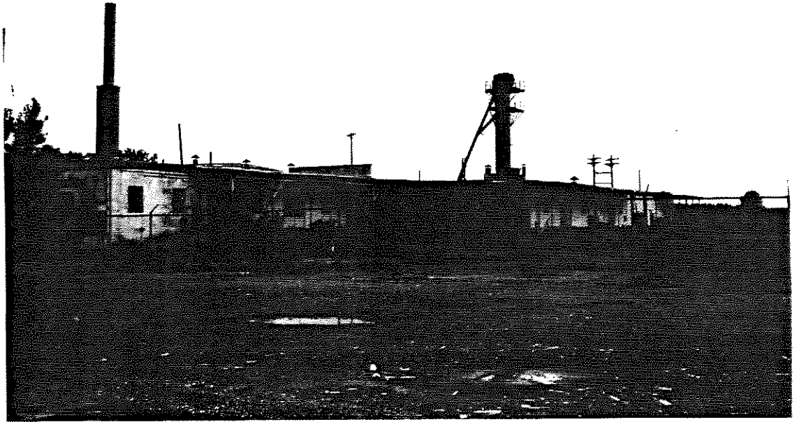
Photo 42: SEAD-16, 9/11/90. View of the Abandoned Deactivation Furnace - Building S-311, facing southeast.
