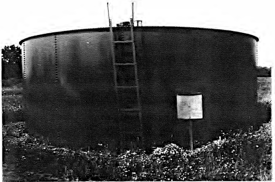
Photo 122: SEAD-50, 9/12/90. View of the Sulfide Ore Tank (Tank No. 17) located at the Tank Farm, facing north.
