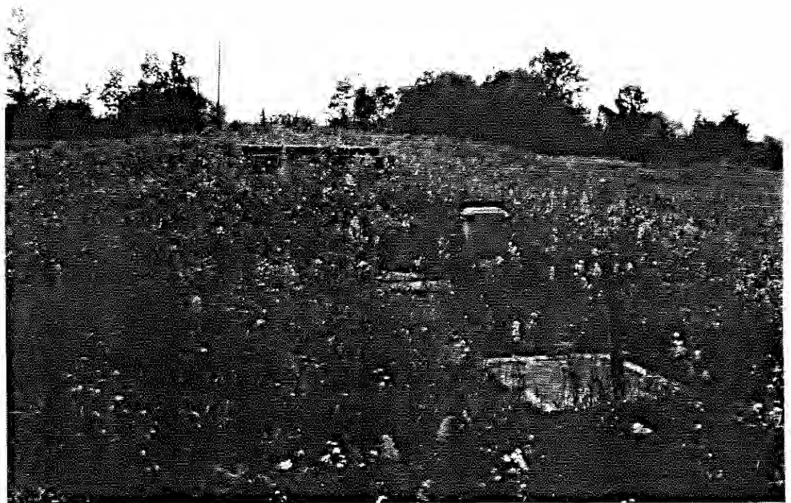
Photo 134: SEAD-56, 9/12/90. View of the septic tank system, Herbicide and Pesticide Storage Area - Building 606, facing south.
