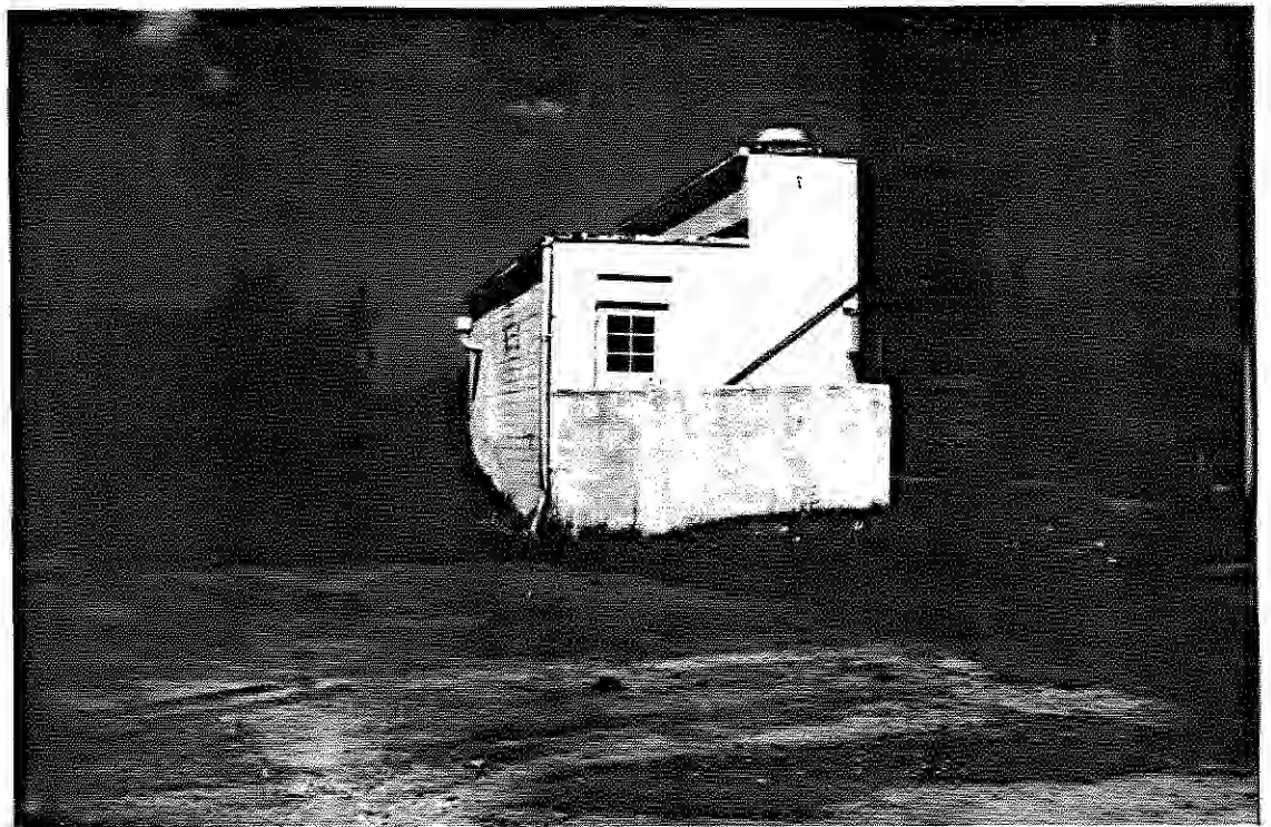
Photo 150: SEAD-60, 9/13/90. View of Oil Discharge - Building 609, facing north.
