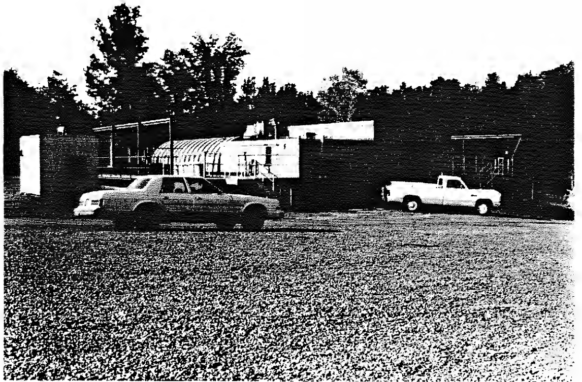
Photo 57: SEAD-21, 9/13/90. View of the Sewage Treatment Plant No.715, facing southwest.
