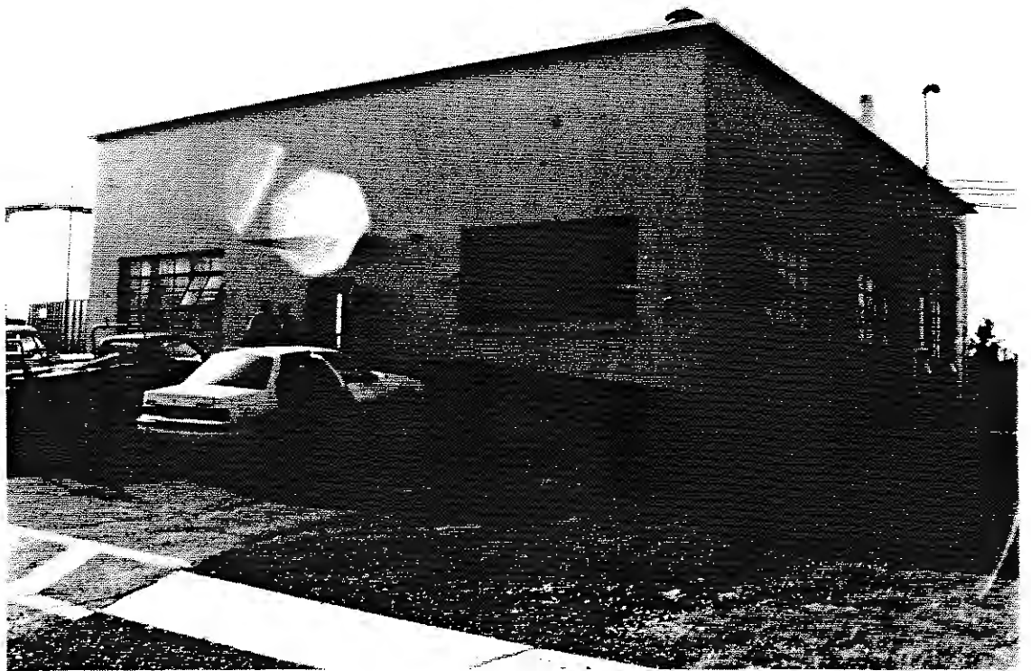
Photo 97: SEAD-35 and SEAD-41, 9/13/90. View of Building 718 where three Waste Oil - Burning Boilers are located, facing south; the Boiler Blowdown Leach Pit (SEAD-41) is located in the vicinity of the building.
