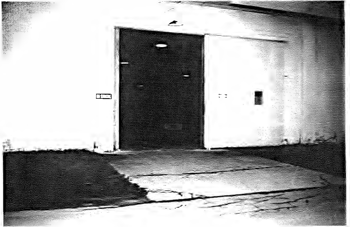
Photo 127: SEAD-55, 9/12/90. View of the Tannin Storage Area - Building 357, facing east.
