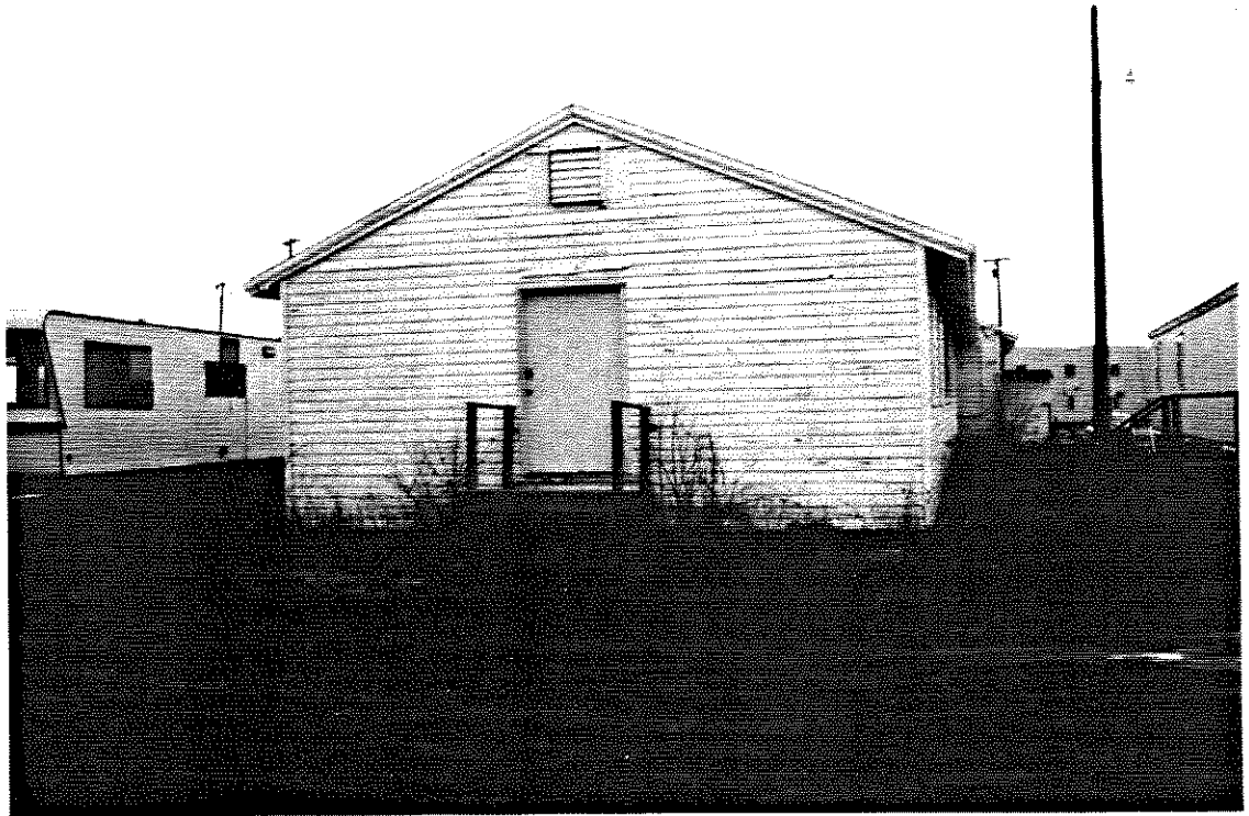
Photo 179: SEAD-68, 11/27/90. View of Pest Control Shop - Building S-335 (Old Firehouse), facing south.
