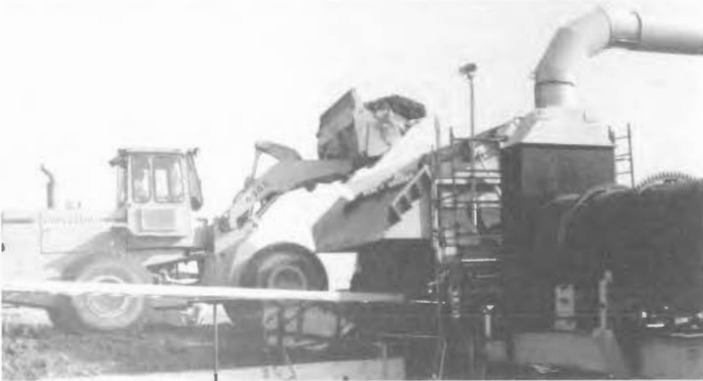
The Marine Corps/Navy treats fuel-contaminated soil at Tustin Marine Corps Air Station using a portable thermal desorption unit.
