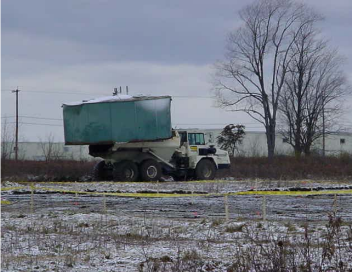
9.) RELOCATING 9,000-GAL ABOVE GROUND STORAGE TANKS TO DISMANTLING AREA
