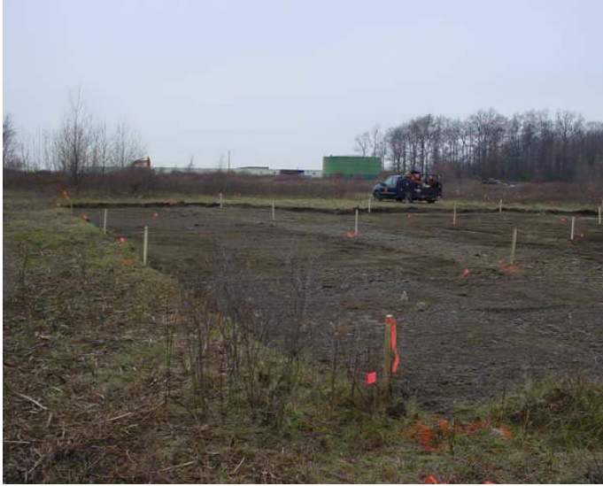
5.) AREA 2 – EXCAVATION, VIEWING NORTHWEST
