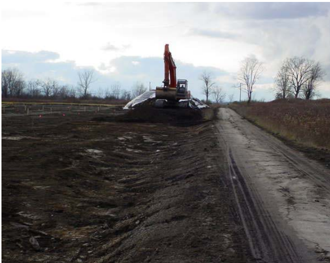
3.) AREA 1 – EXCAVATION, VIEWING WEST ALONG PAVED HAUL ROAD
