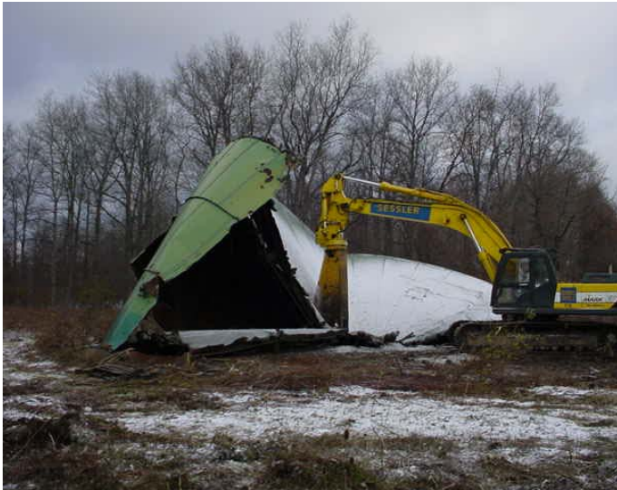
7.) 507,000-GAL ABOVE GROUND STORAGE TANK BEING DISMANTLED WITH HYDRAULIC SHEARS
