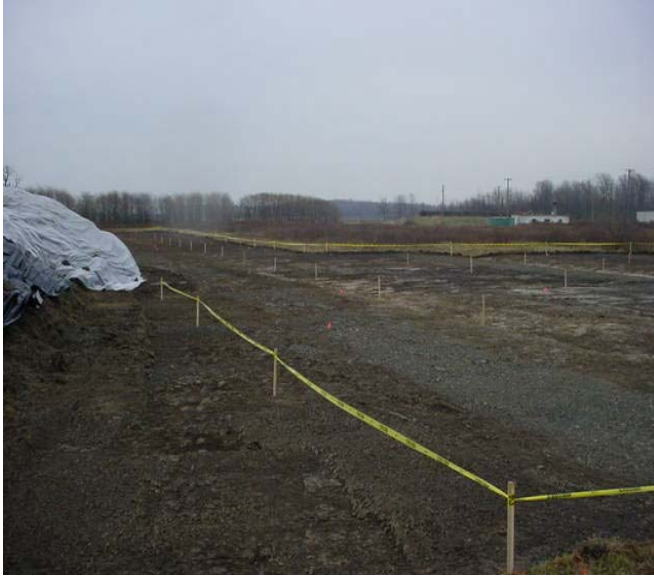
1.) AREA 1 – EXCAVATION TO A DEPTH OF 6-INCHES, VIEWING EAST
