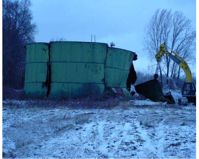
6.) 507,000-GAL ABOVE GROUND STORAGE TANK BEING DISMANTLED WITH HYDRAULIC SHEARS
