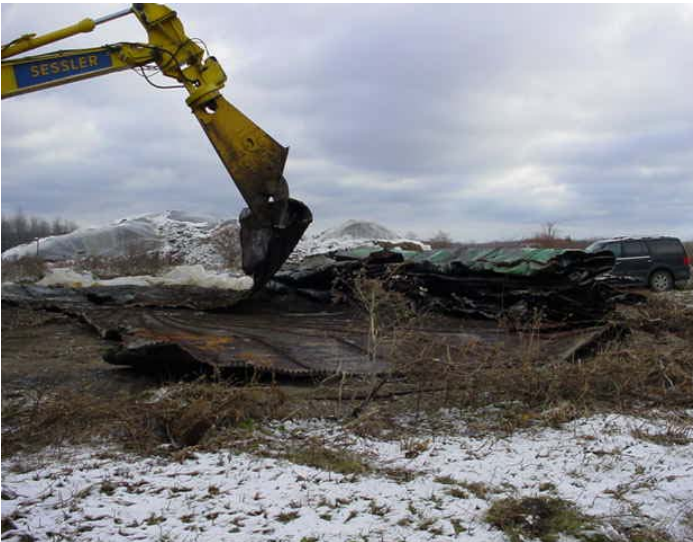
11.) STEEL FROM ABOVE GROUND STORAGE TANKS ROLLED UP FOR T&D
