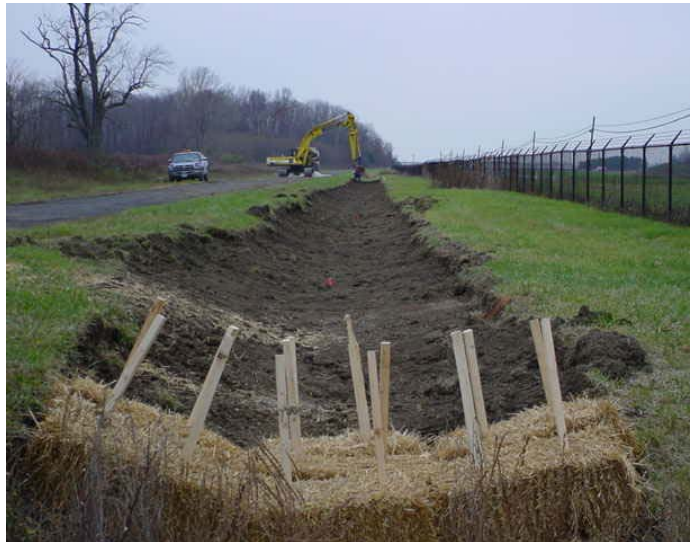
12.) AREA 7 – VIEWING NORTH ALONG THE EXCAVATION LIMITS
