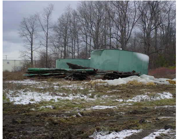
8.) 507,000-GAL ABOVE GROUND STORAGE TANK FOLDED INTO MANAGEABLE SECTIONS
