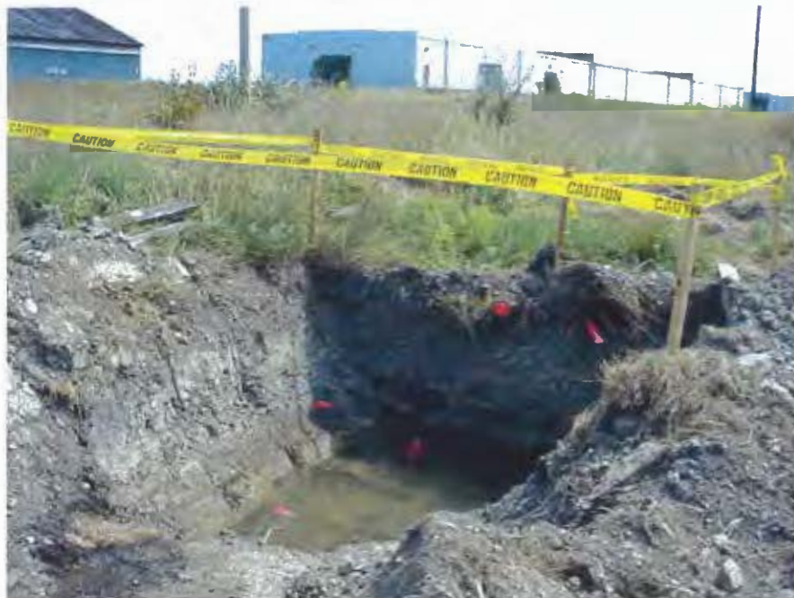
Photograph #4- View of the northern portion of the ditch with 6-ft excavation at SEAD 40.
