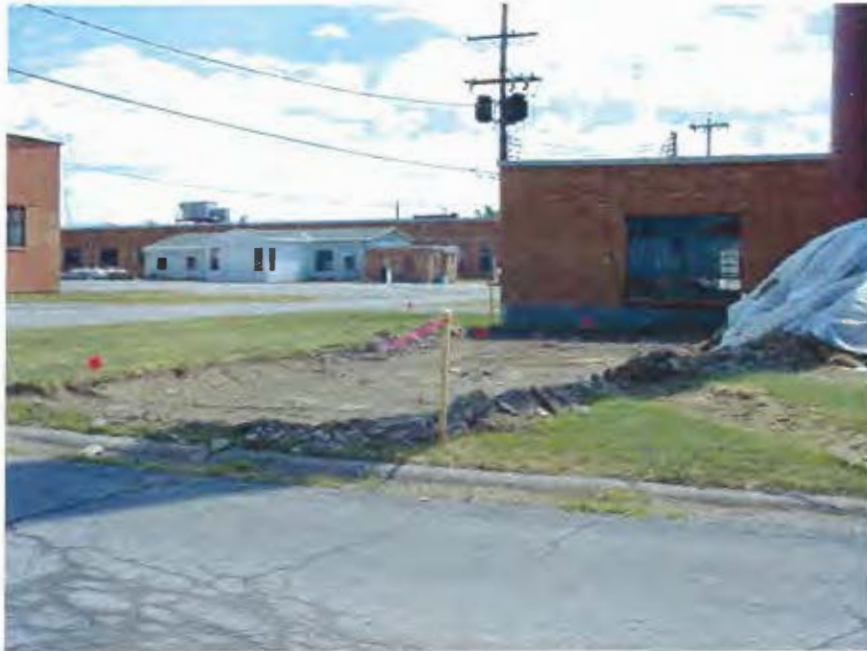
Photograph #1 – View of the excavation area adjacent to Building 121 at SEAD 39.
