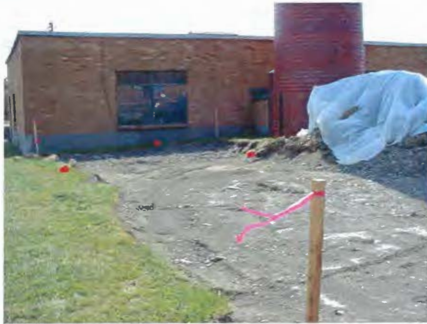
Photograph #3 - Top six inches of clean soil was excavated and staged on site for future backfill at SEAD 39.
