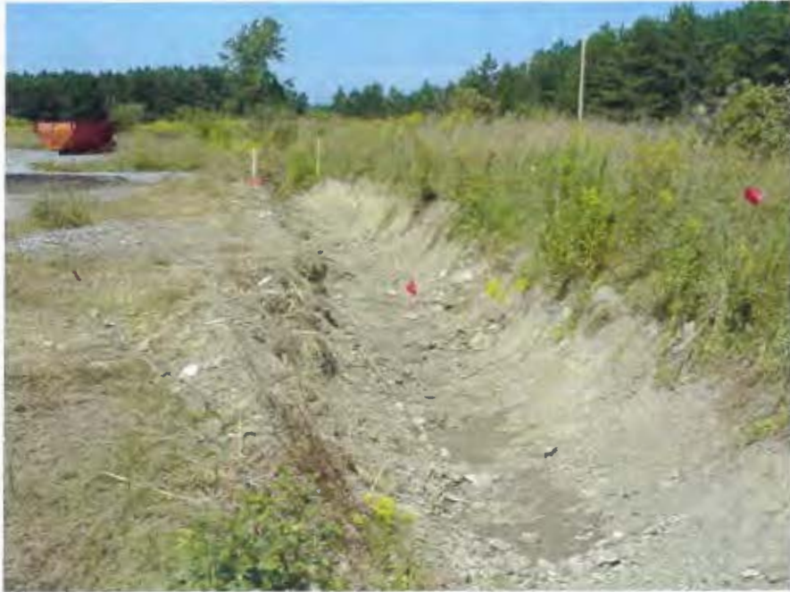
Photograph #5 - View of the excavated trench with one-foot excavation at SEAD 40.
