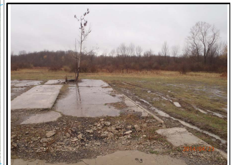
Status as of: 4/23/14 Photo ID: P4230196.JPG Description: SEAD-17, Building 367 foundation.
