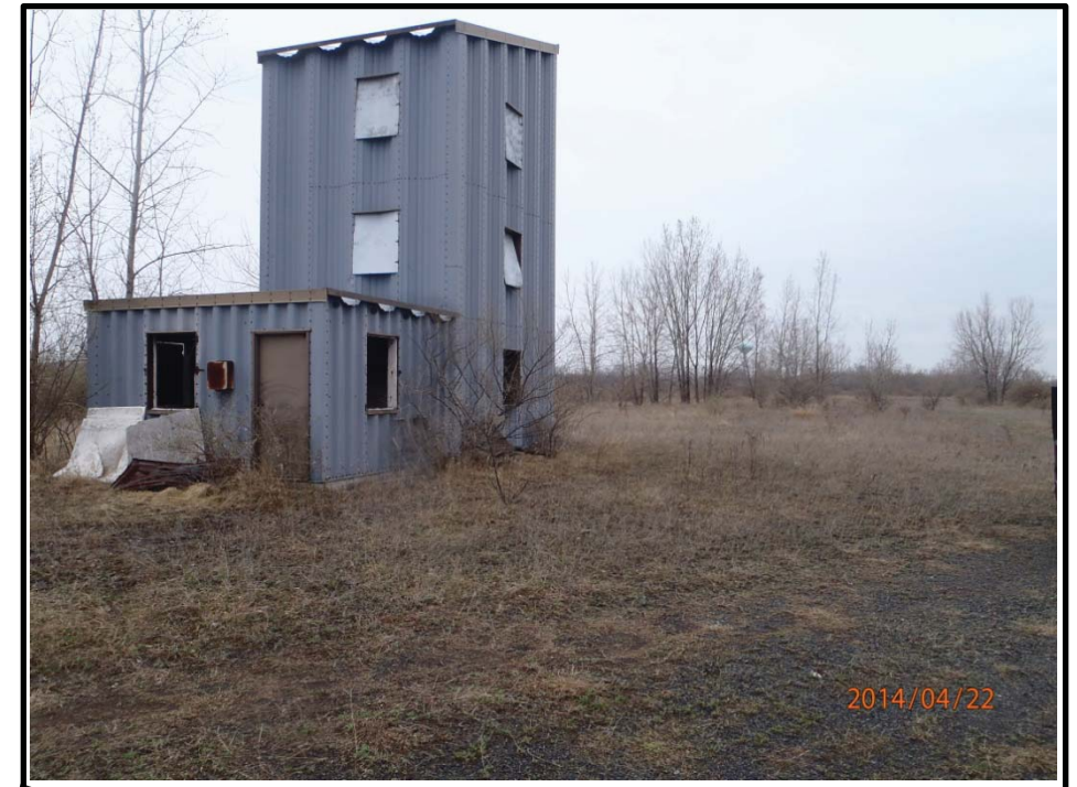
Status as of: 4/22/14 Description: SEAD-26
