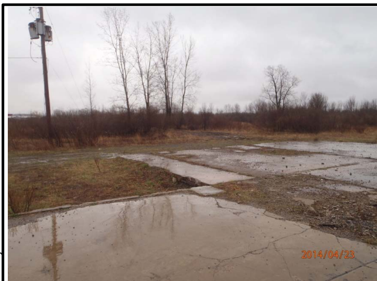
Status as of: 4/23/14 Photo ID: P4230195.JPG Description: SEAD-17, Building 367 foundation.
