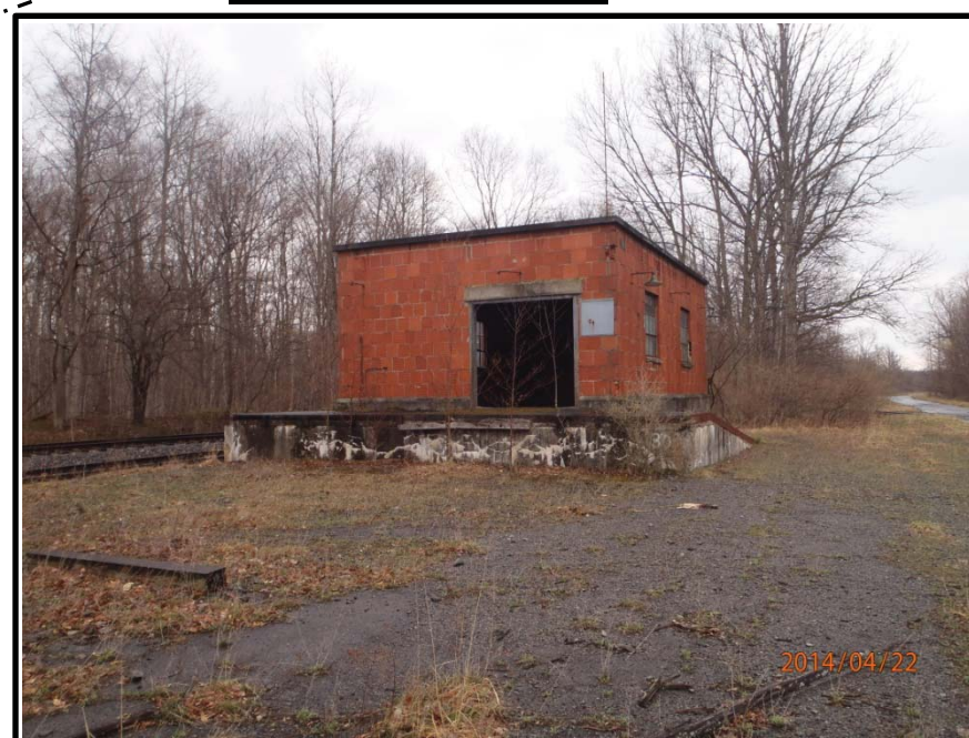
Status as of: 4/22/14 Description: Building 307
