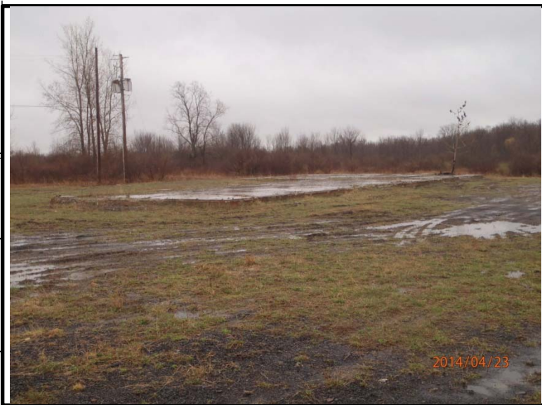
Status as of: 4/23/14 Photo ID: P4230198.JPG Description: SEAD-17, Building 367 foundation.
