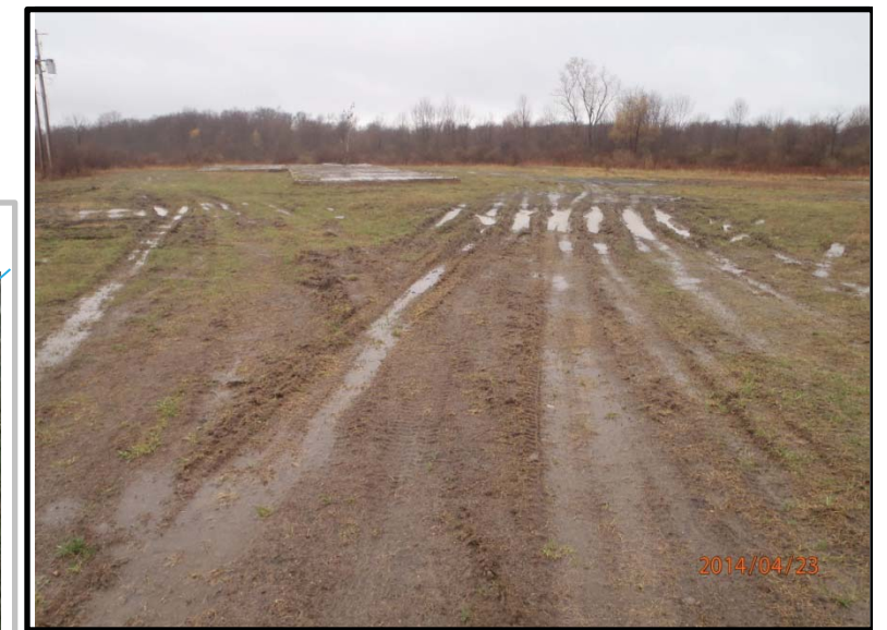
Status as of: 4/23/14 Photo ID: P4230194.JPG Description: SEAD-17, Building 367 foundation.
