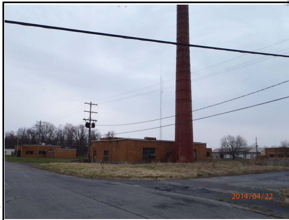
Status as of: 4/22/14 Photo ID: P4220003.JPG Description: SEAD-39 blowdown pit in foreground
