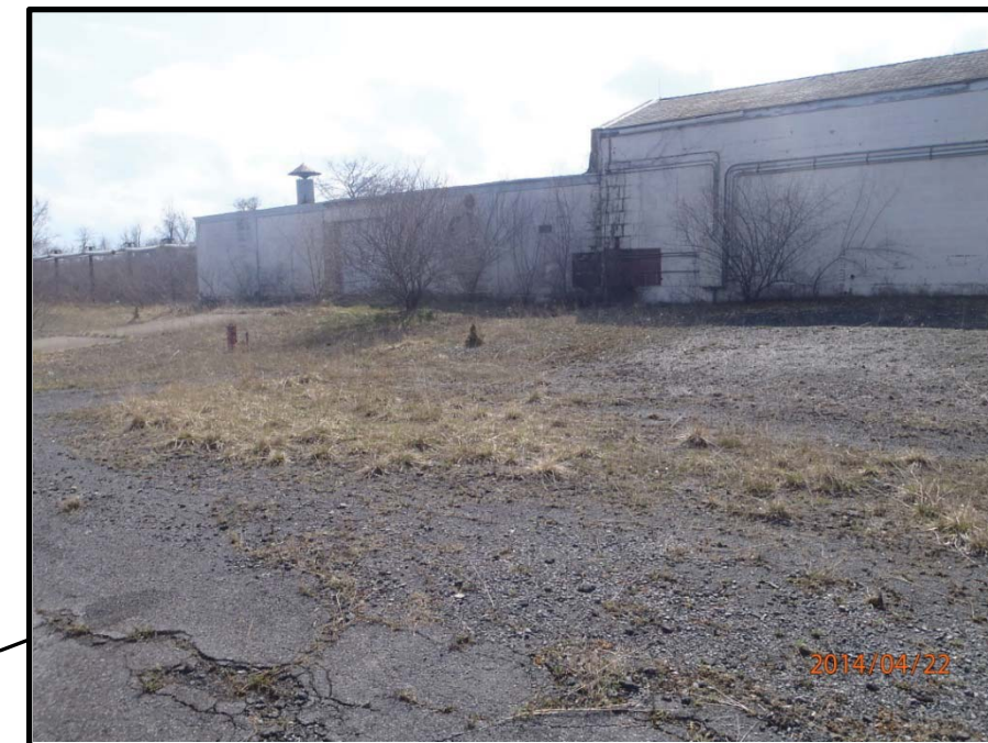
Status as of: 4/22/14 Description: SEAD-40
