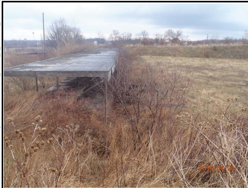
Status as of: 4/22/14 Description: SEAD-122B Photo ID: P4220116.JPG
