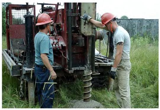
Status as of: 7/9/02 Description: View of drillers collecting spilt-spoon samples during the drilling of monitoring well MW-2. Photo by: EJA
