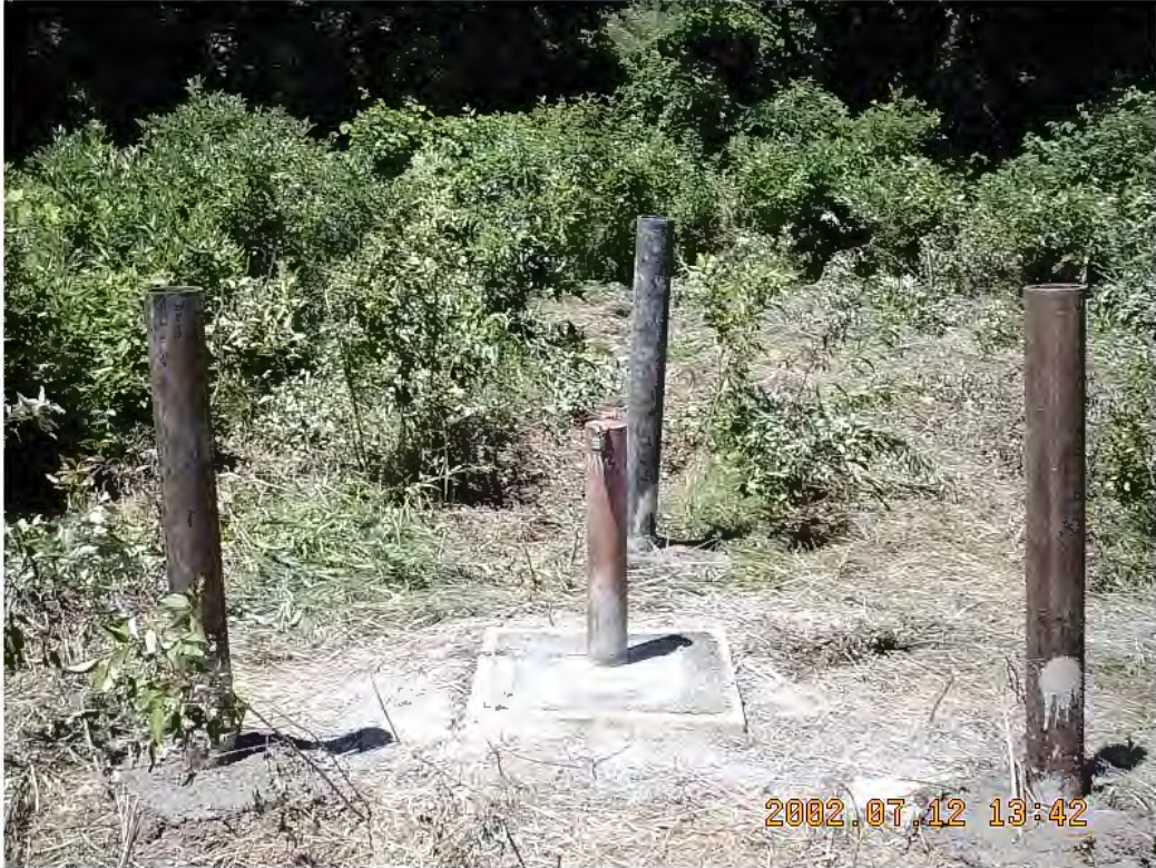
Status as of: 7/9/02 Description: View of monitoring well MW-1 after installation completed. Photo by: EJA
