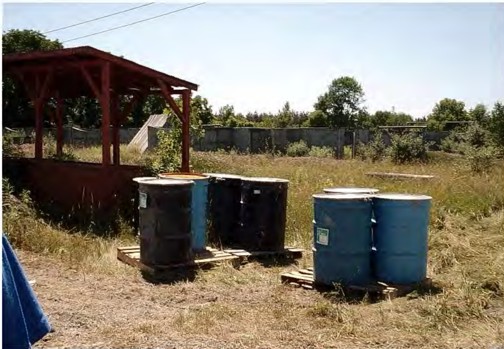
Status as of: 7/9/02 Description: View of IDW contained in 55-gallon DOT drums staged onsite (SEAD-122B) on wooden pallets. Photo by: EJA
