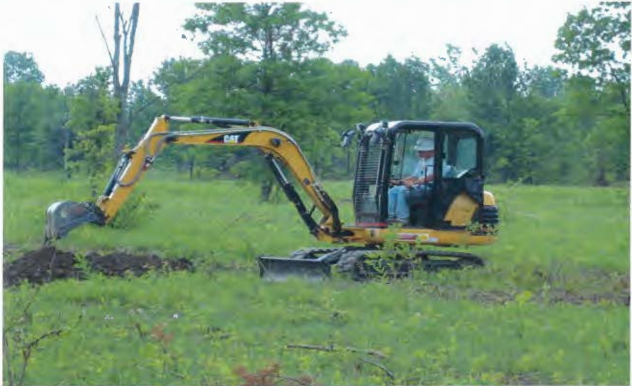
Photo No. 6: Placing USACE QA Seed Items Using a Mini-excavator
