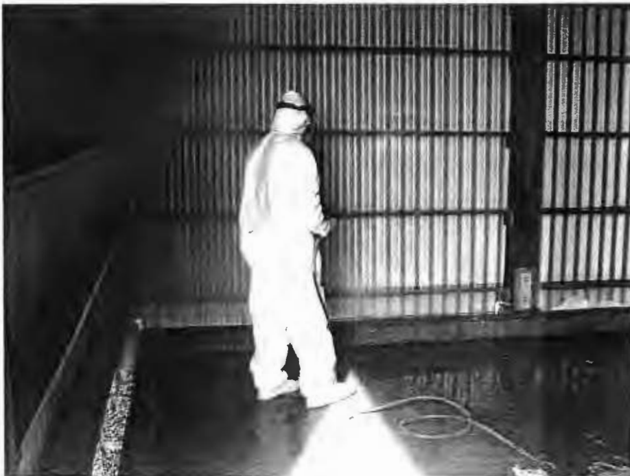
Washing inside of Bldg 307.
