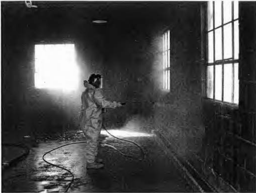
Performing cleaning operations at Bldg 301.
