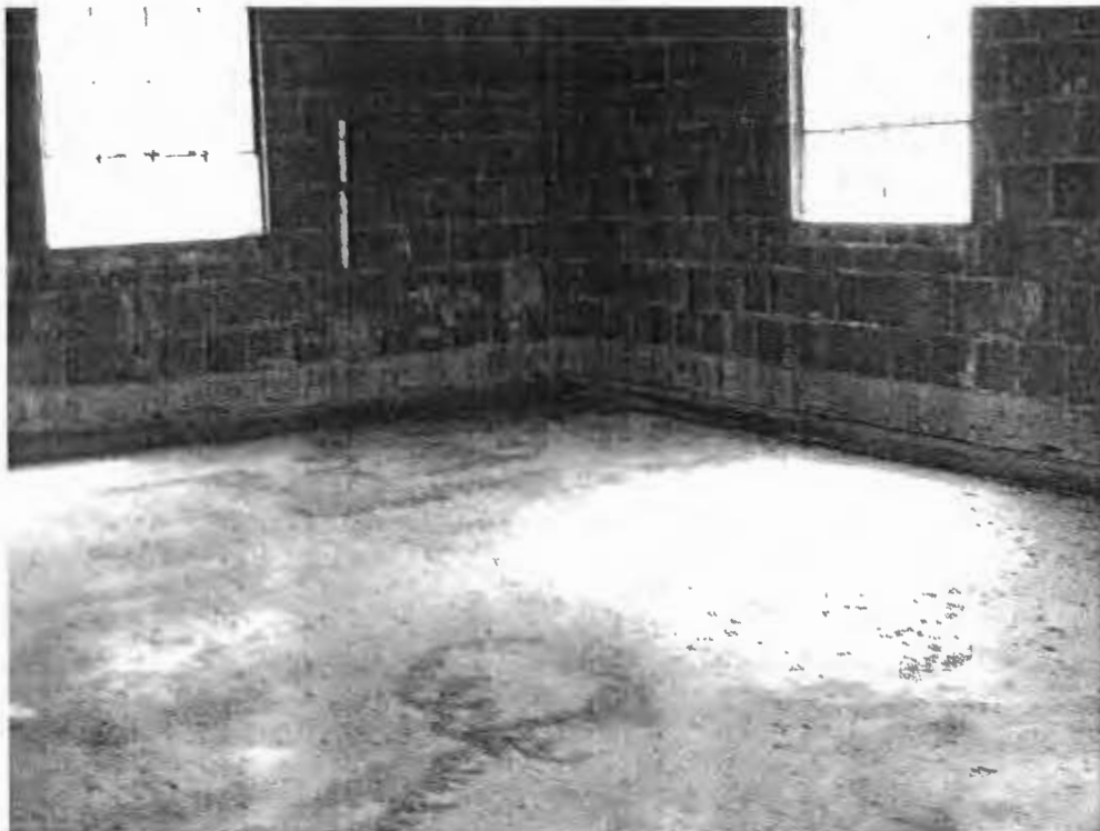
Building 301 after debris removal.
