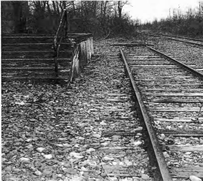
Location of railroad bed adjacent to building.
