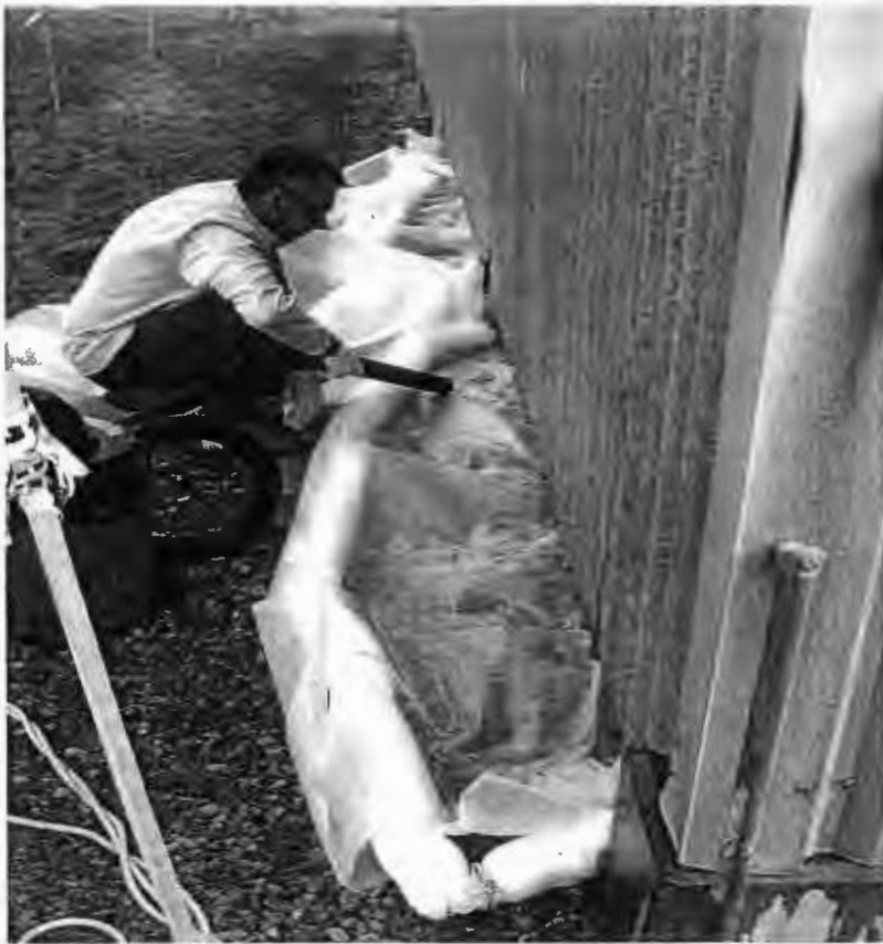
Collecting rinsate from wall washing
