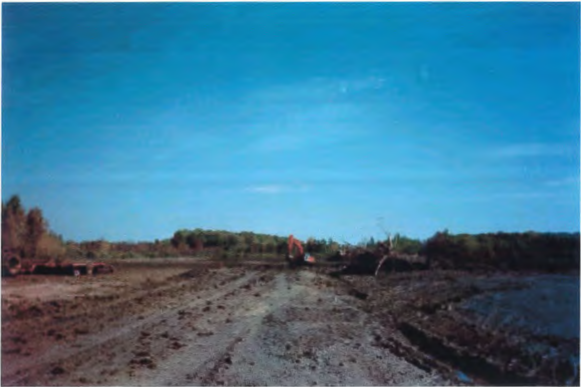
Figure G-13 Draining water for the site.
