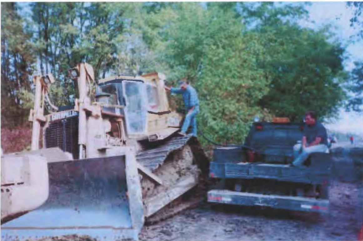
Figure G-22 Subcontractor servicing excavation equipment.
