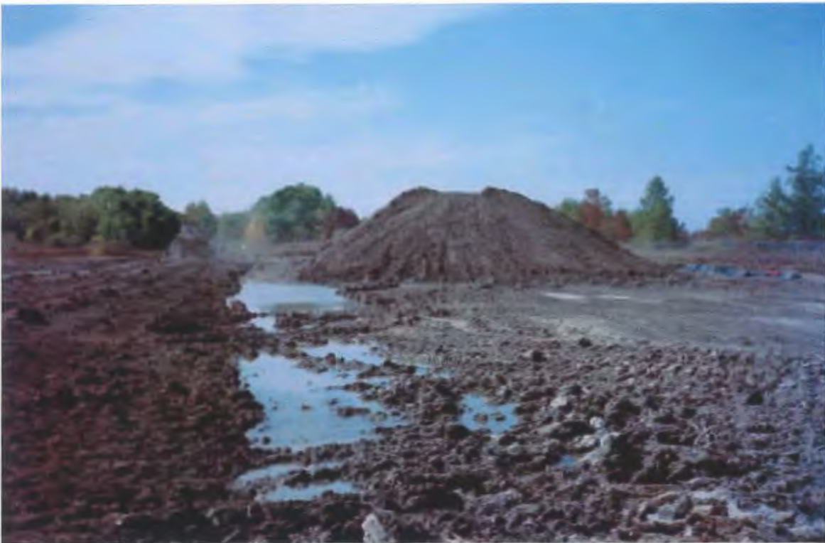
Figure G-20 Material to be sifted.
