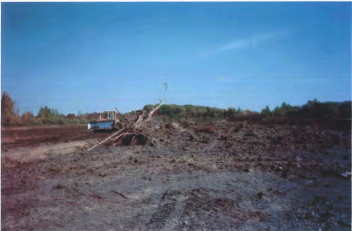
Figure G-18 Clearing vegetation.
