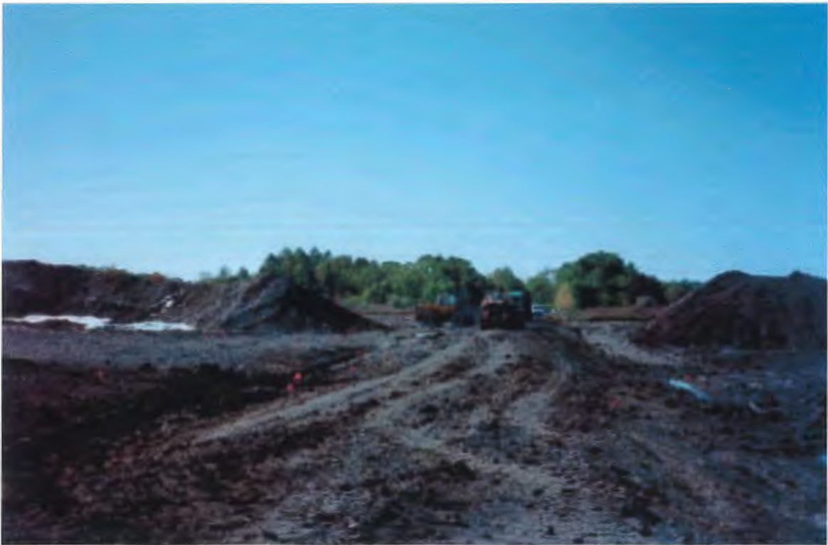
Figure G-4 Soil being laced into drying piles.
