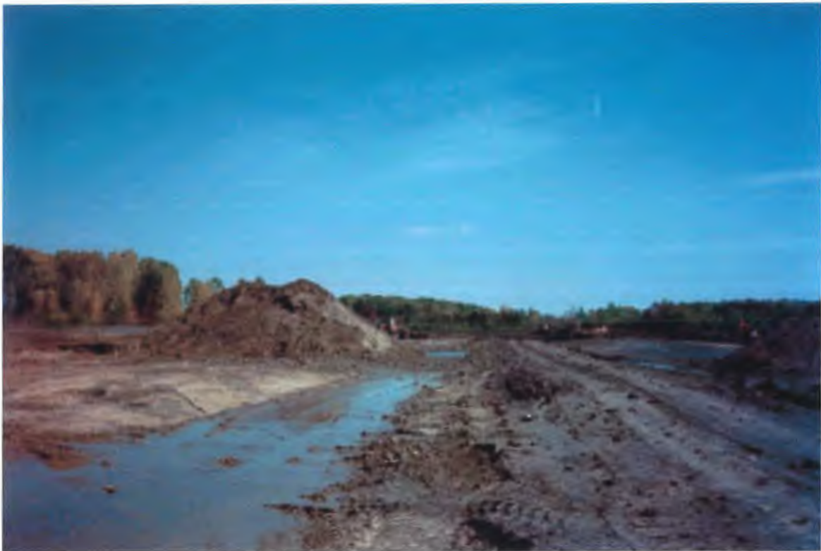
Figure G-10 East view from gate area.
