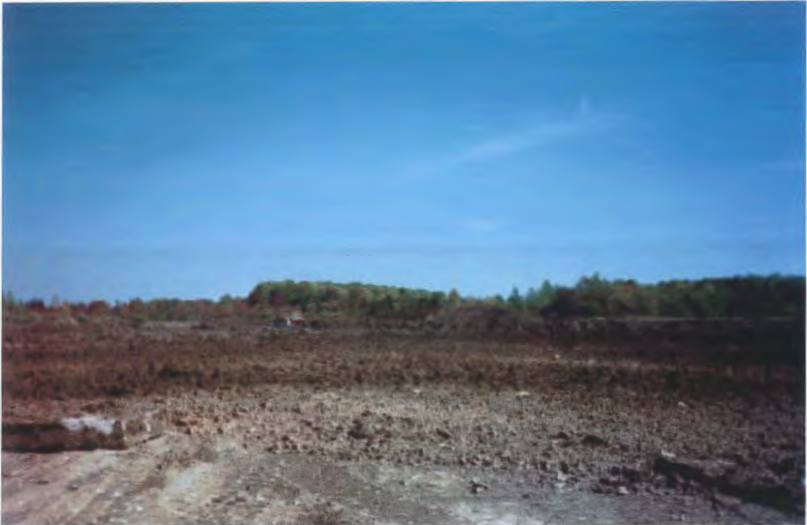
Figure G-17 Piling soil to be sifted
