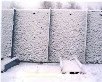
21. Emergency shield outside emergency exit for UXO technicians. Material made of two pieces of 5/8" steel
