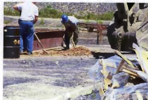
31. Loading OE Material into burn cage
