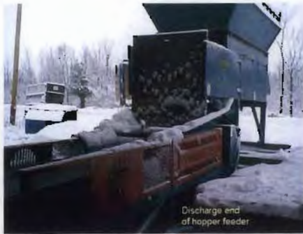
15. Discharge end of conveyor hopper
