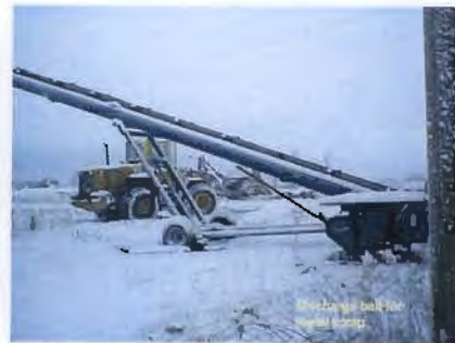
22. Discharge belt for metal scrap
