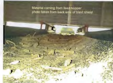
26. View from back side of blast shield
