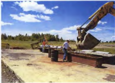
32. Using excavator to place burn cage on dunnage
