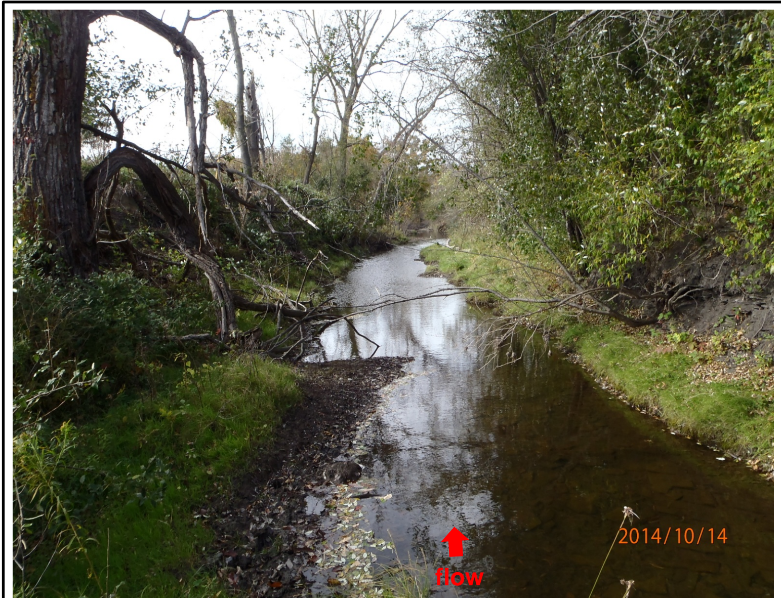
Photo #17 – Looking northwest (downstream) in Reeder Creek. Each side of the creek is well vegetated. Fractured shale and brown slime observed along the creek bottom.
