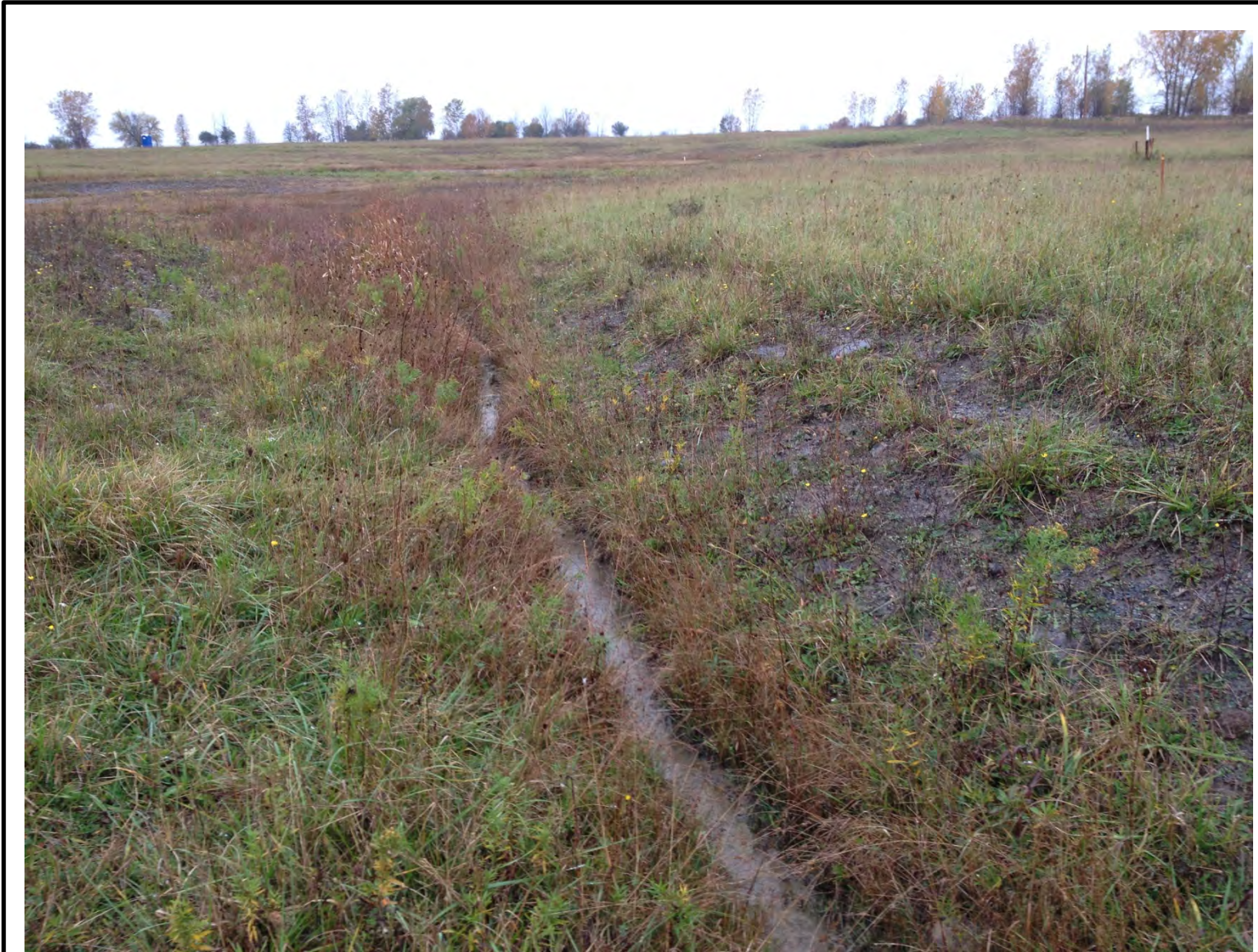
Photo #05 – Grid I8. No erosion or disturbances observed. Well vegetated. Drainage ditch operating as intended. View to the west.
