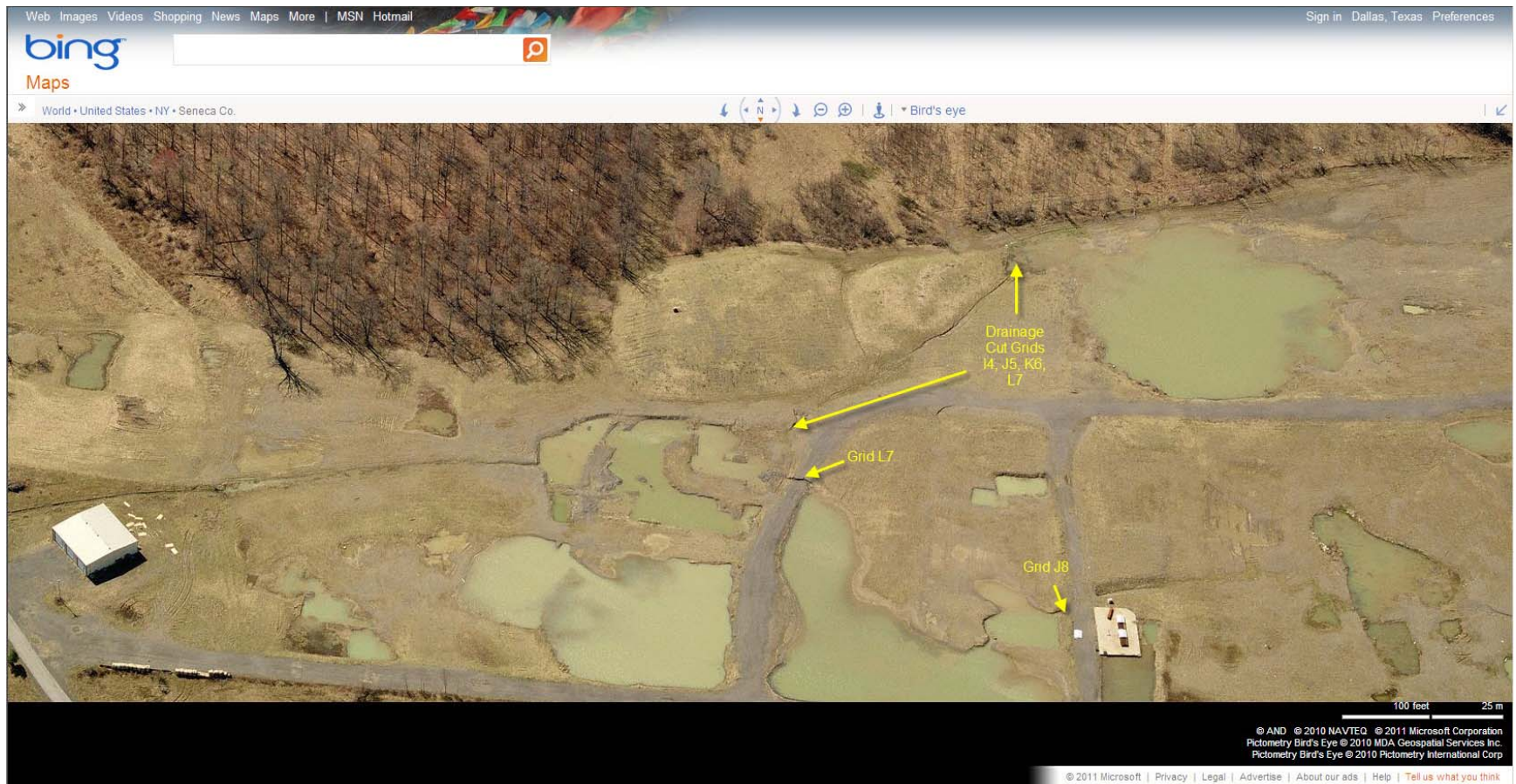
Figure 13 Aerial View of OB Grounds with Approximate Locations of August 2010 Inspection Comments Identified
