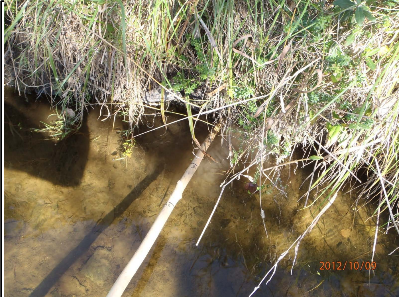
Photo #19 – Looking at west embankment (OB/OD Side) of Reeder Creek. Approximately 12 inches of creek bank have been scoured out along the embankment;.
