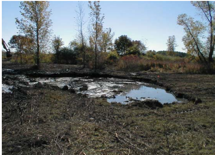
Northwest Debris Pile (SEAD-14) excavated - looking west.
