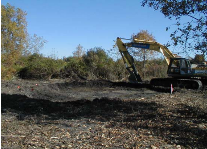
Southwest Debris Pile (SEAD-14) excavated - looking south.
