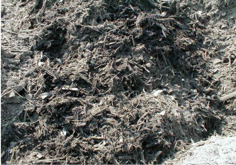
Mulch/Sand Mixture in Trench
