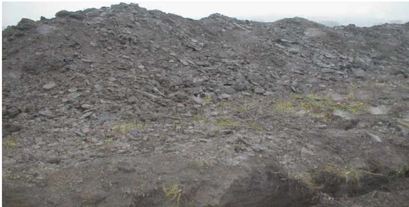
C2 trench spoils. Note the shale removed to get to bedrock.
