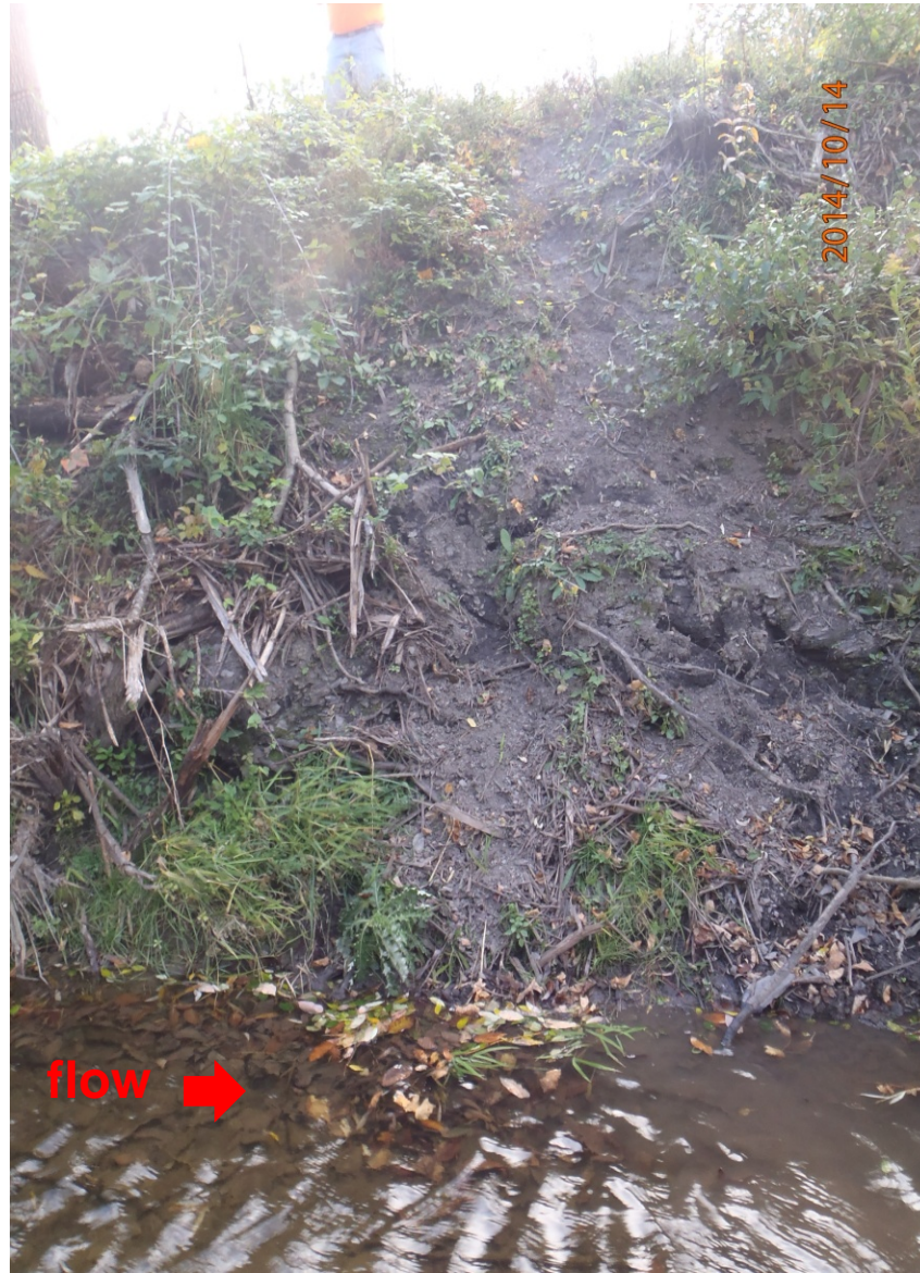
Photo #15 – Looking at the west creek embankment (OB grounds side) of Reeder Creek. Local erosion is present; however, no evidence present of overland flow occurring or excessive deposition of sediment into the creek.
