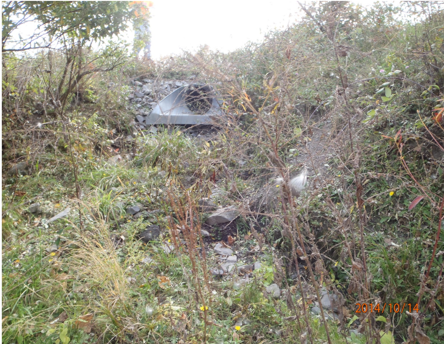
Photo #45 – Looking southwest at the culvert on the OB grounds side of creek. No evidence of washout leading from culvert down into the creek.
