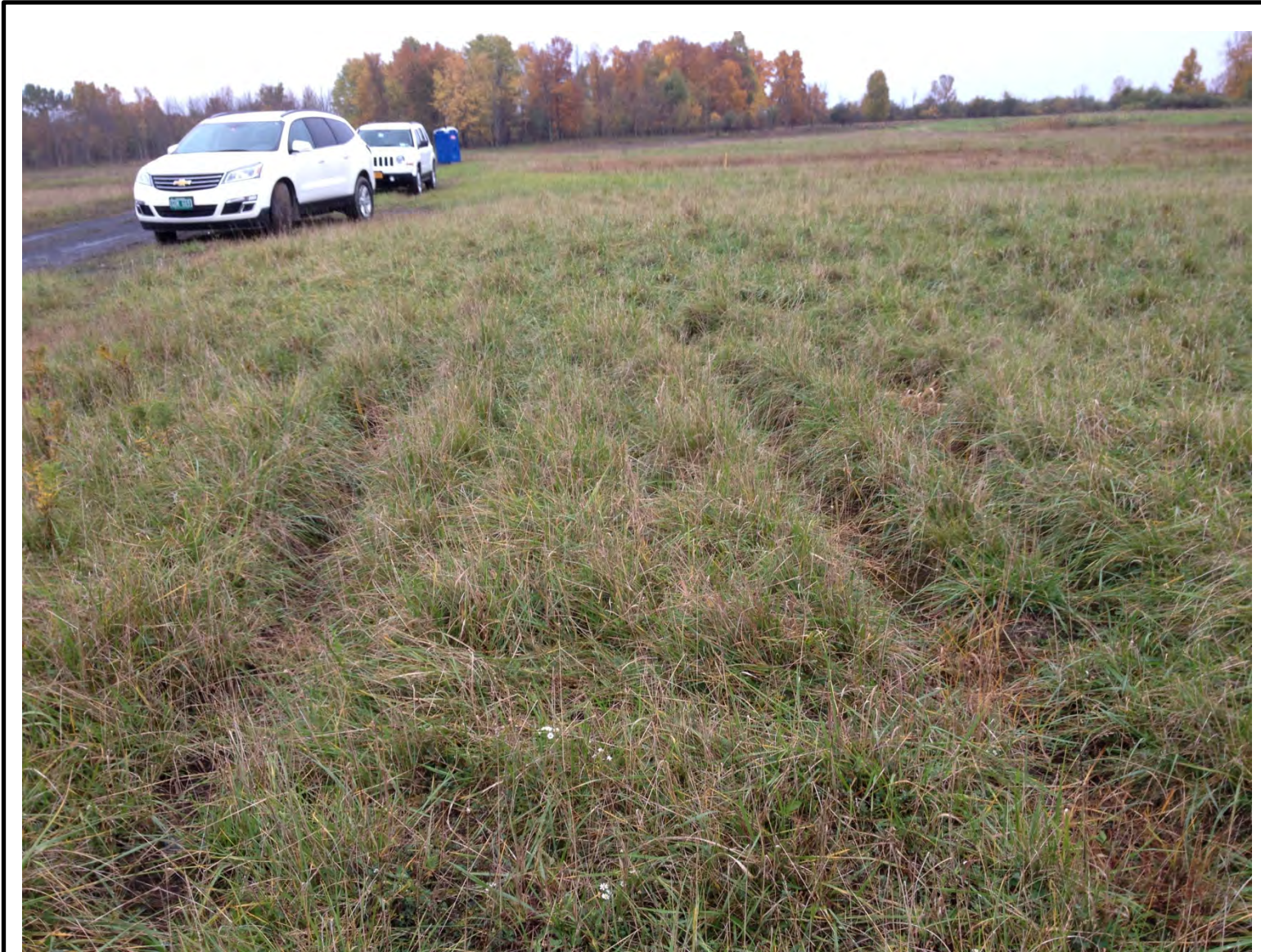
Photo #03a – Grid C7. No erosion observed. Well vegetated. Several tire ruts ranging from 3-10 feet long and 2-6 inches deep. View to the south.
