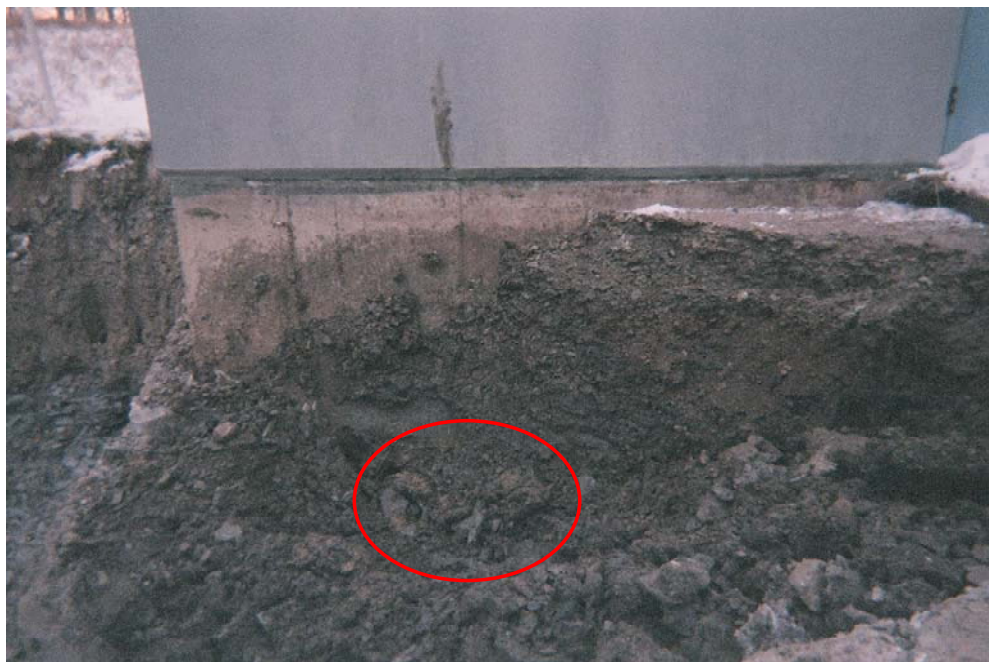
Remains of 4-inch Ductile Iron pipe
