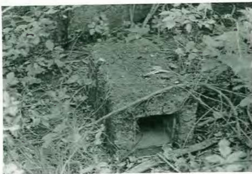
Figure 26. Photograph of chimney fragment at site A09906.000164.
