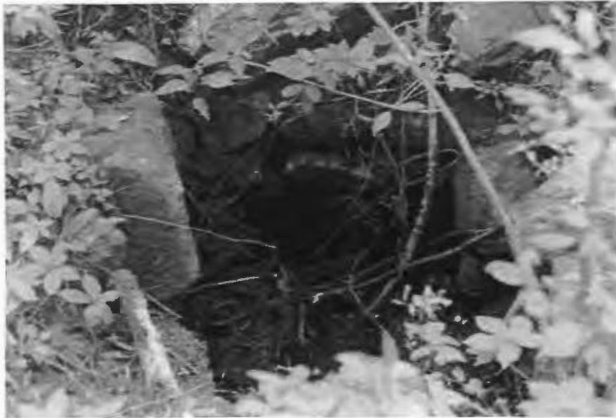
Figure 29. View of a portion of the rock-lined foundation at site A09906.000166.
