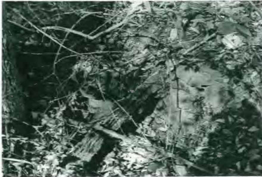
Figure 86. Collapsed rock-lined well at site A09906.000201/A09906.000234.
