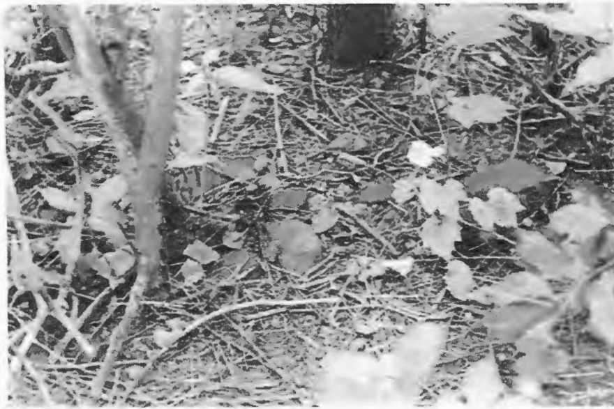
Figure 151. View of a portion of the remnant stone foundation at site A09909.000019.
