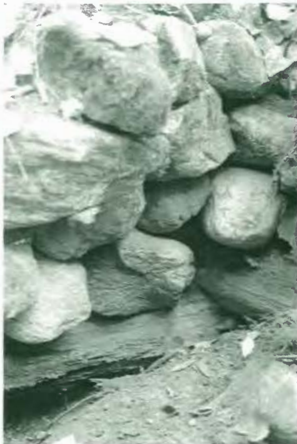
Figure 192. View of the log and rock construction of the wall in the pit-like feature.
