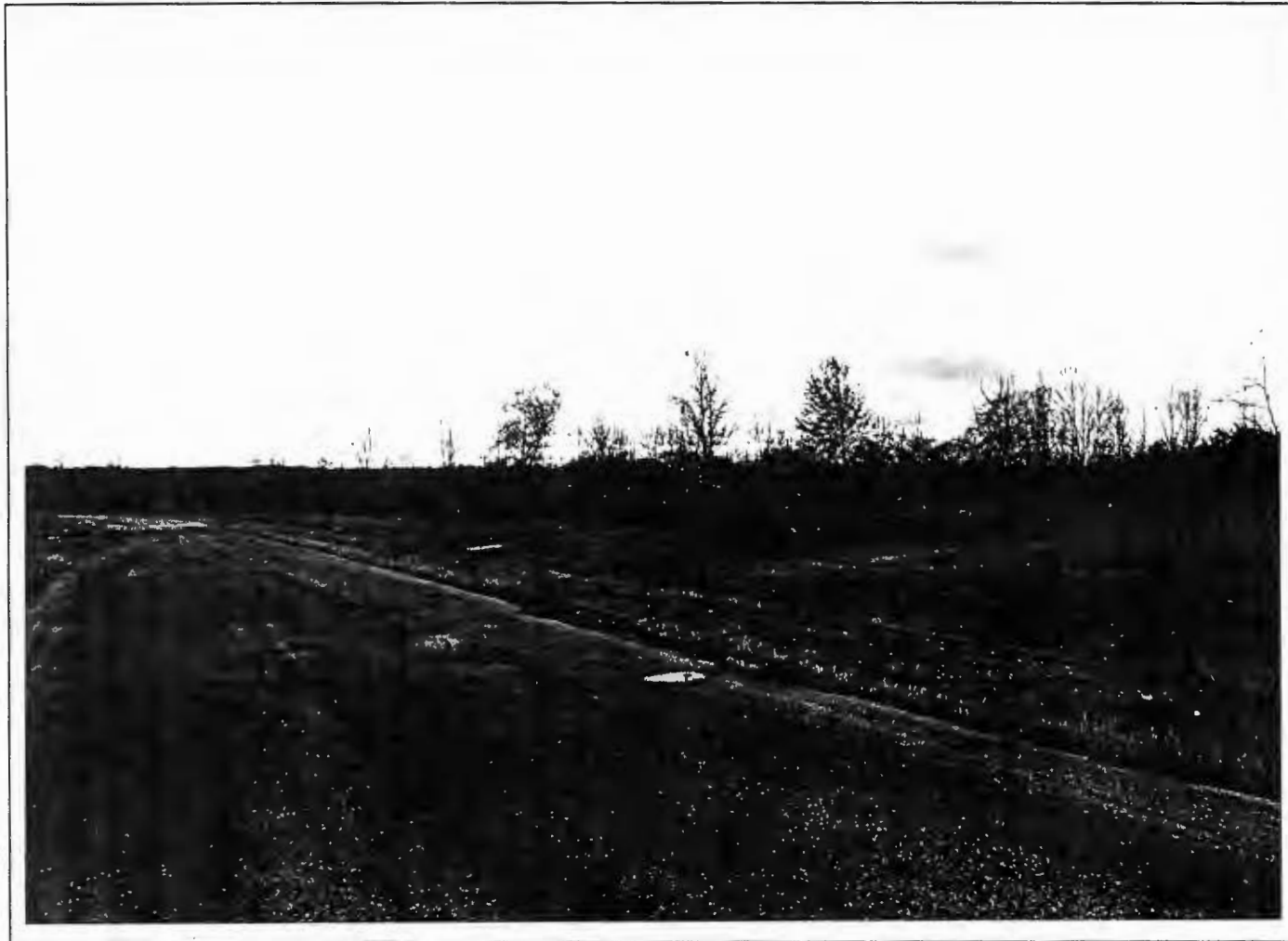
Figure 5-14. Poorly drained area off Seneca Road, west of Washout Facilities in Area 2, drainage ditches in foreground. Seneca Army Depot Activities, Seneca County, NY.
