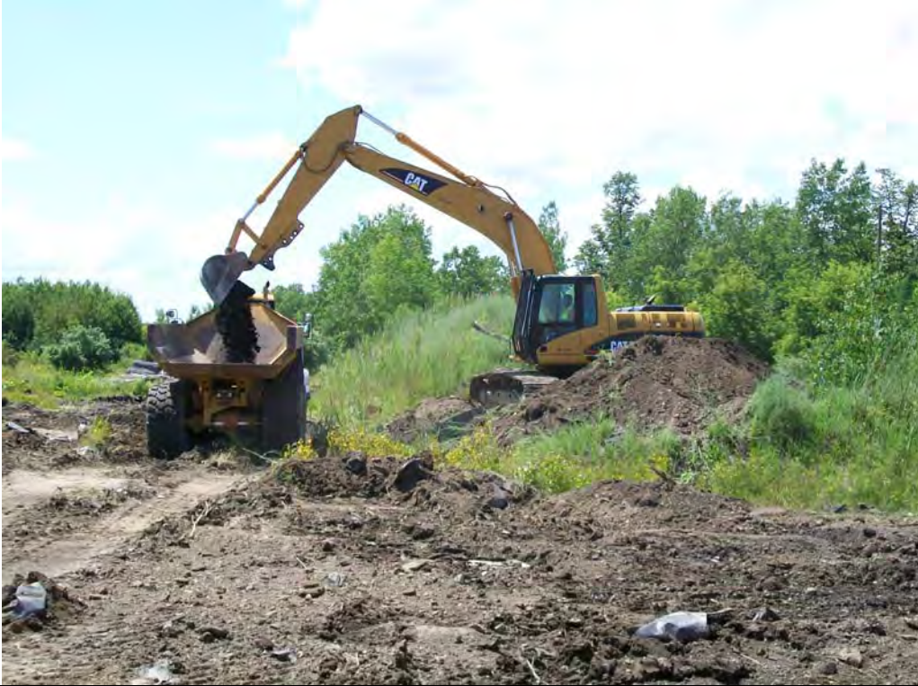
Photo: 7 Date: 7/6/2009 Site: SEAD-59 Description: Excavator loading haul truck with material from the SEAD-59/71 North Staging stockpiles.
