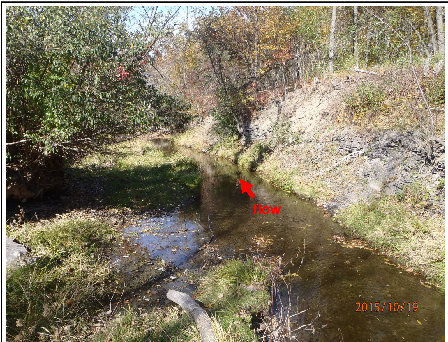
Photo #2 – Looking northwest (downstream). Vegetated embankments (east and west) on each side of Reeder Creek. Water levels in the creek are low, similar to the 2014 inspection.
