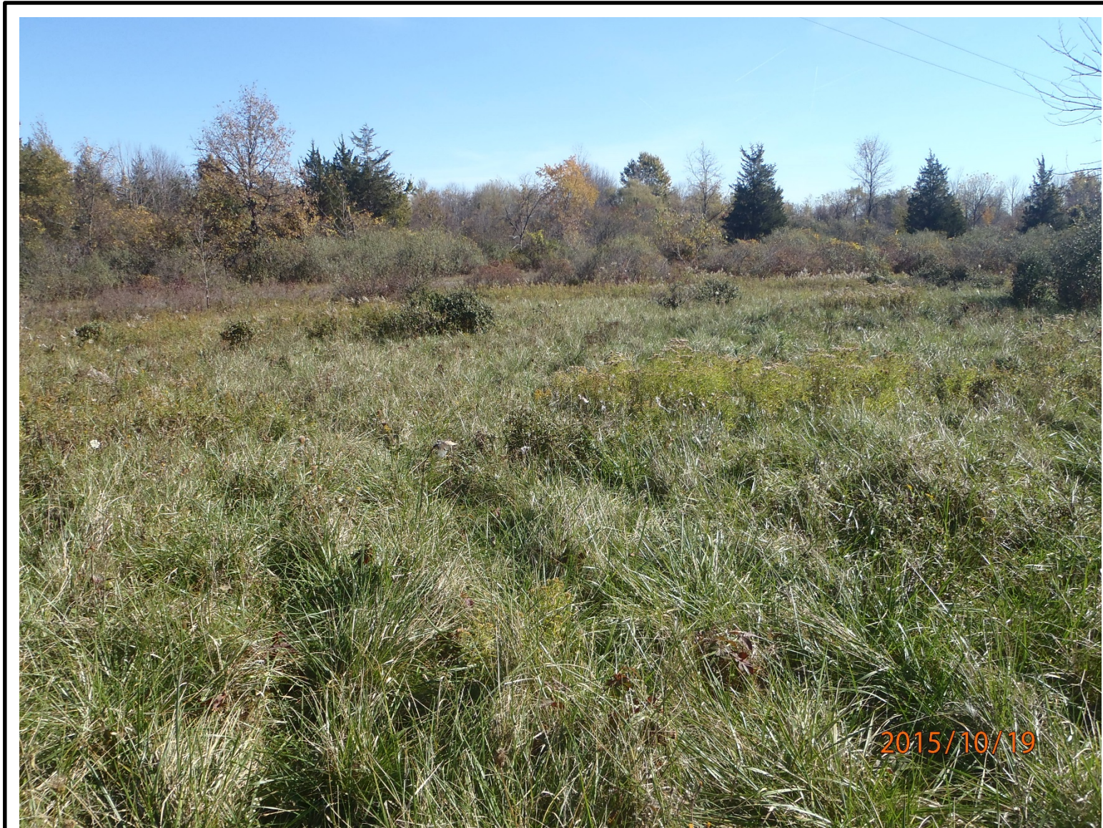
Photo #03 – Grid S8. No erosion or disturbances to the cap were observed. The grid is very well vegetated. View to the east.
