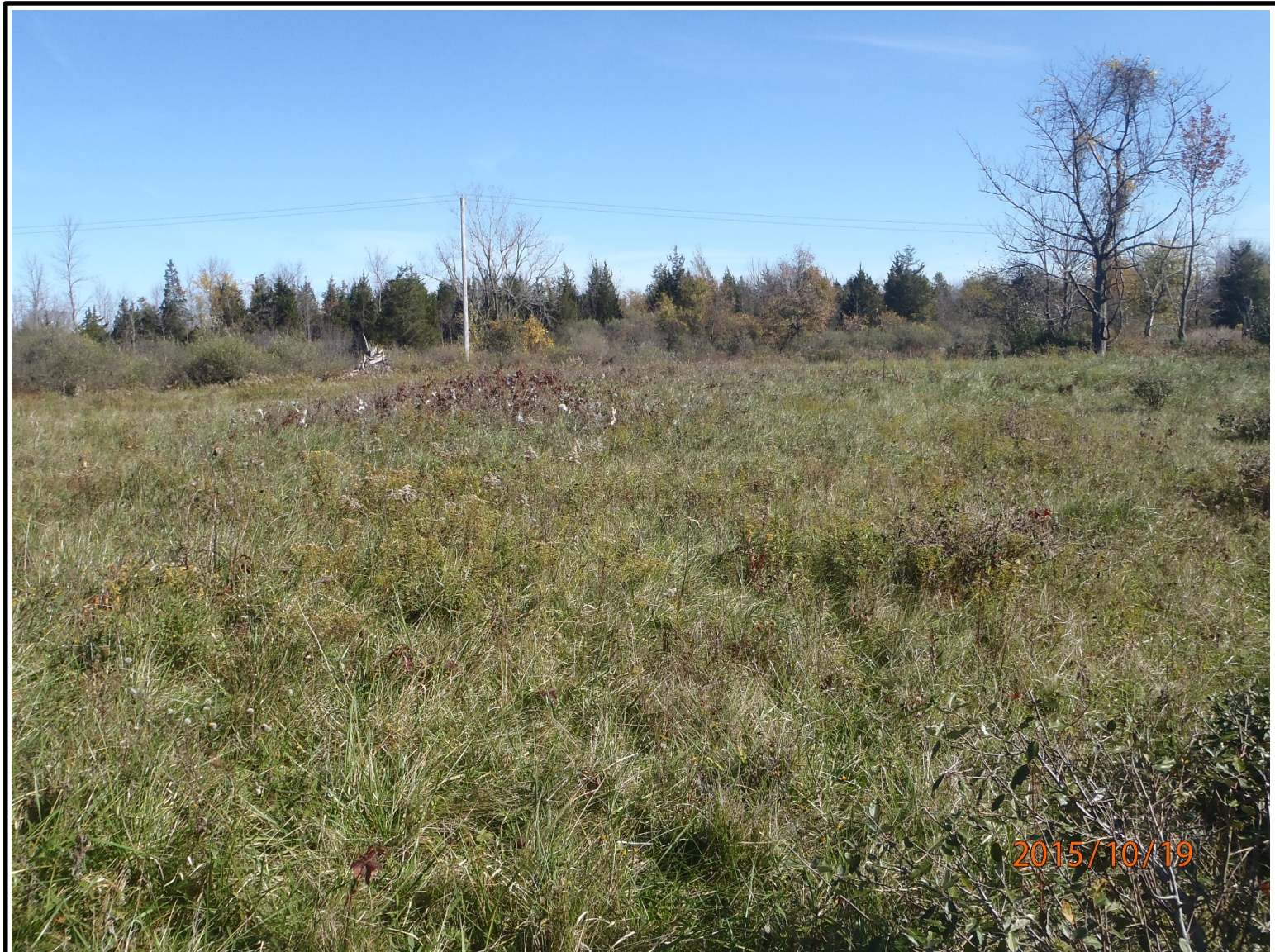
Photo #02 – Grid R8. No erosion or disturbances to the cap were observed. The grid is very well vegetated. View to the east.
