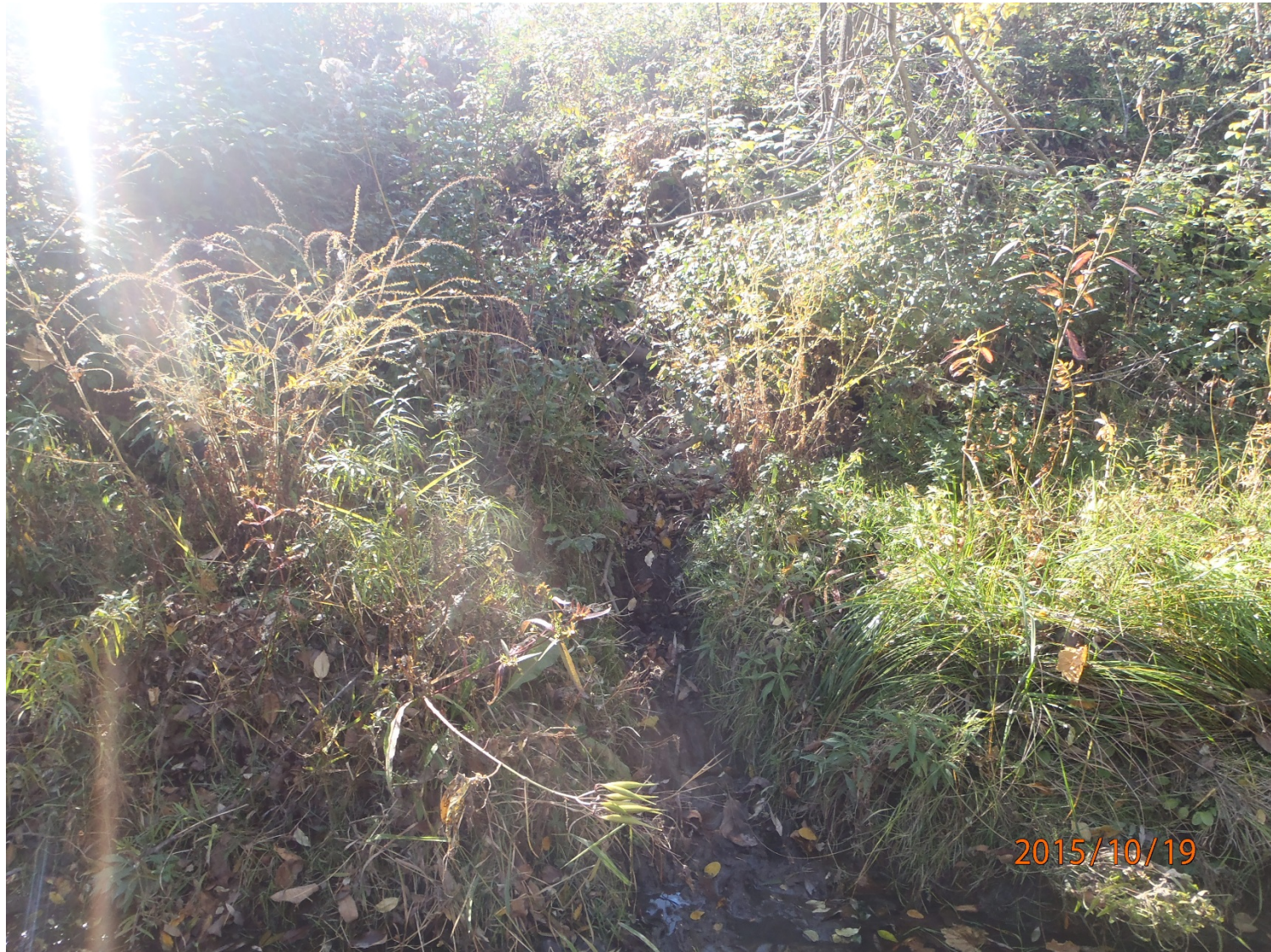
Photo #21 - Looking southwest at creek embankment on the OB grounds side of Reeder Creek. Embankment is well vegetated with apparent deer trail leading down to the water's edge. No evidence of overland flow depositing sediment into the creek.
