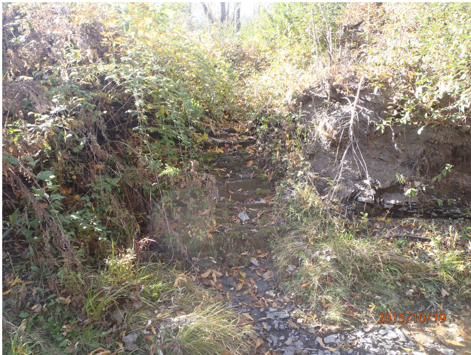
Photo #5 – Looking west at the embankment on the OB Grounds side of Reeder Creek. The embankment is steeply sloped with vegetation and apparent deer tracks leading down to the water's edge.
