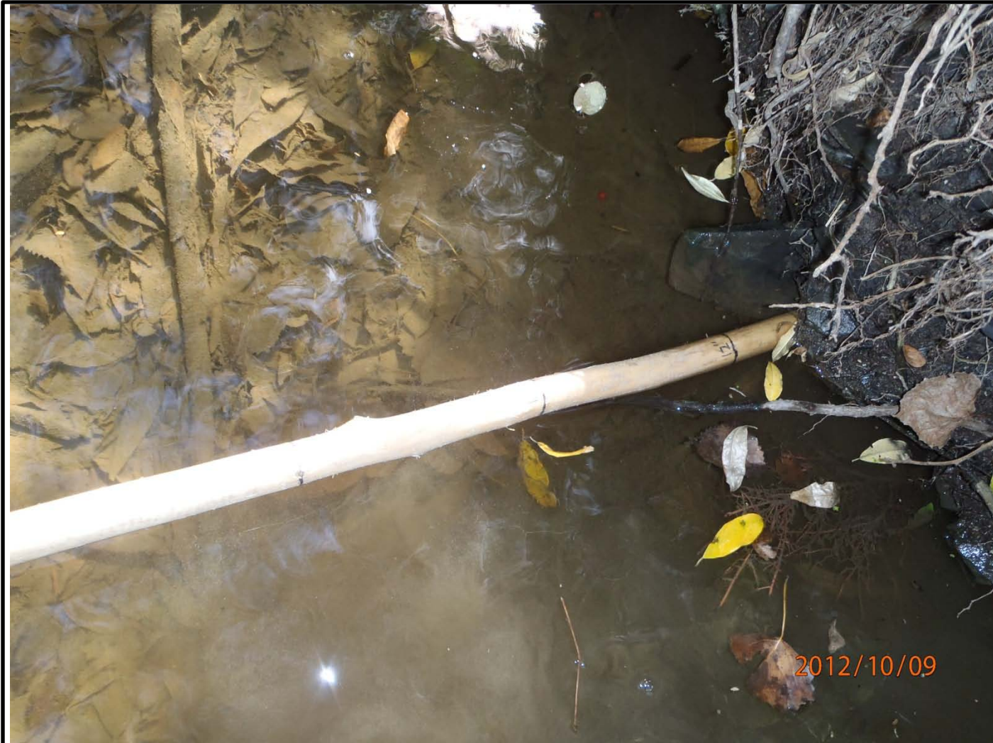
Photo #25 -- Looking at west embankment (OB/OD Side) of Reeder Creek. Approximately 10 inches of creek bank have been scoured out along the embankment;. Accumulation of fallen leaves and branches visible on creek bottom.
