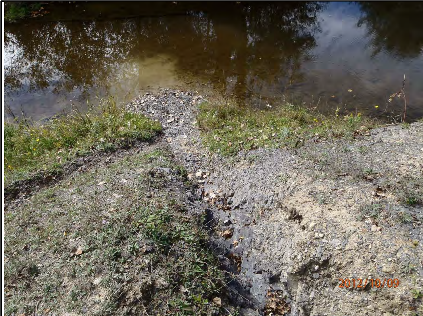
Photo #30 – Looking from on top of the east (SEAD-12) embankment of Reeder Creek. Embankment composed of shale layers with thin vegetated layer. Deer trails to creek are visible in photo. Deer trails cut into embankment 6-10 inches.
