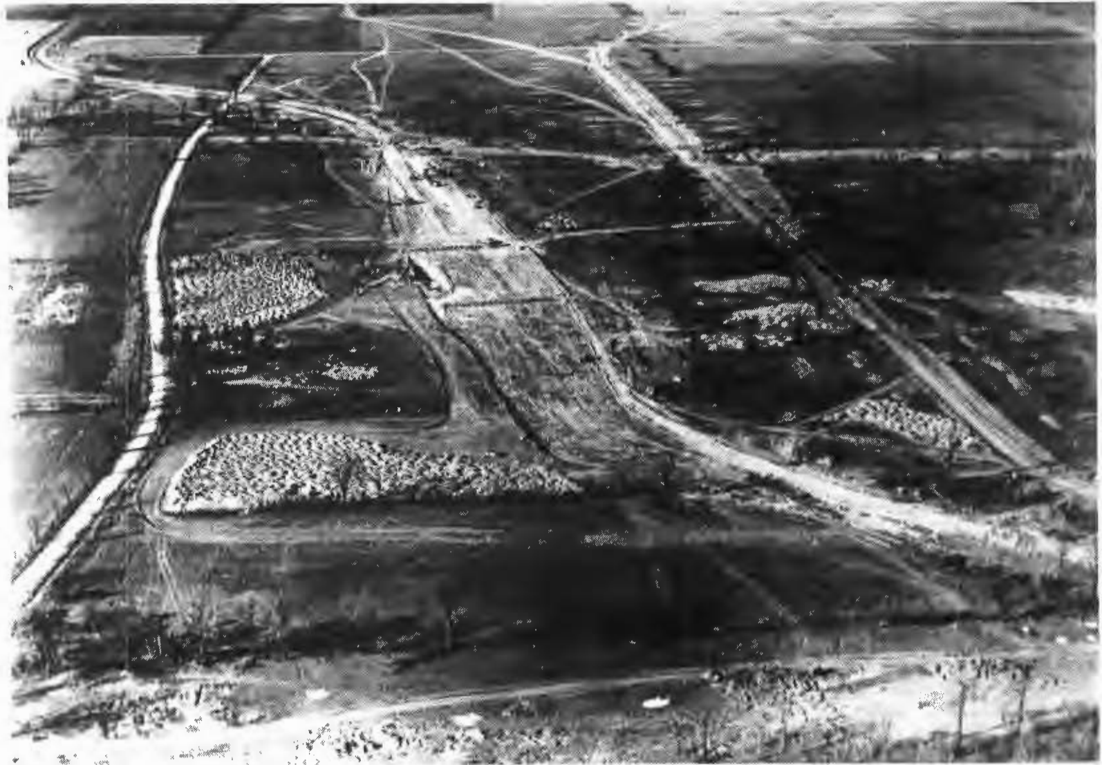
Figure 10. Construction of Classification Yard, facing west.
