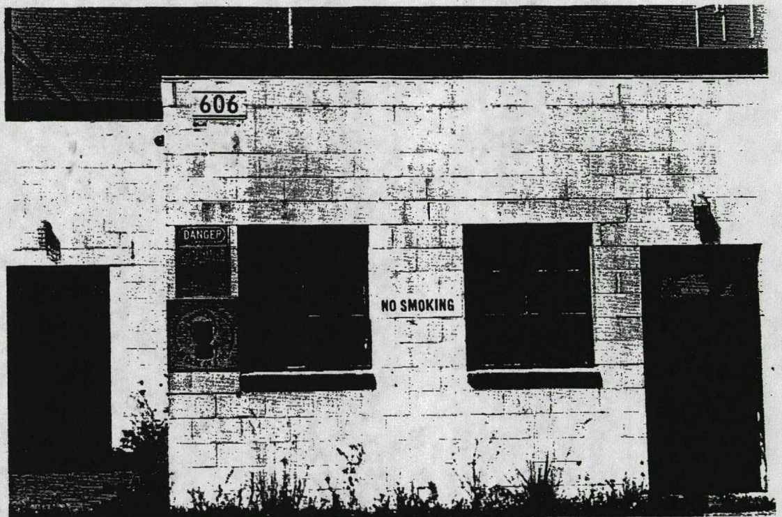
Photo 130: SEAD-56, 9/12/90. Close-up of the signs posted on the Herbicide and Pesticide Storage Area, facing north.
