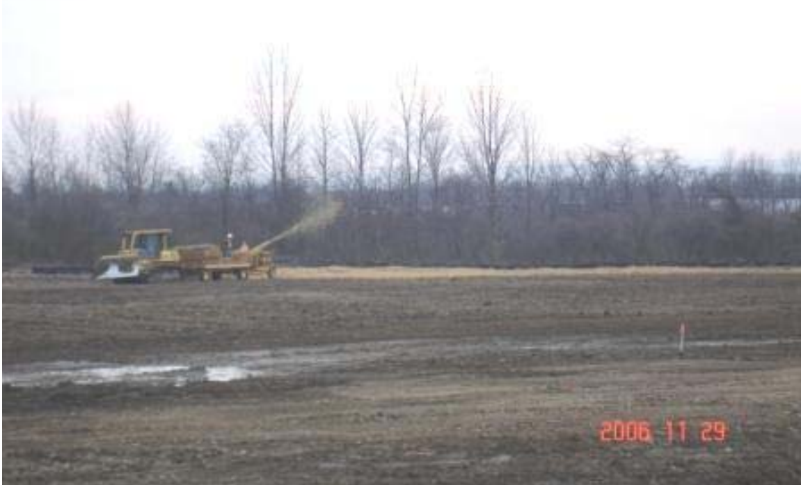
Loc: SEAD-11 Photo#: 19 Date: November 29, 2006 Desc: Establishment of seeding and mulch cover
