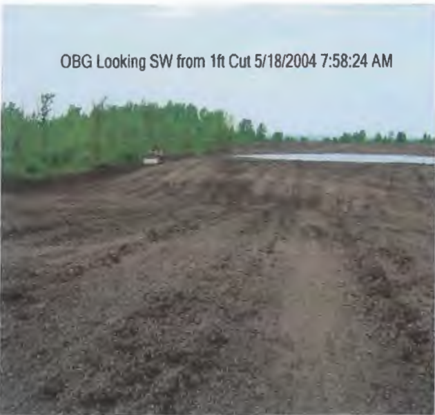
OBG Looking SW from 1ft. Cut at Grid K5
