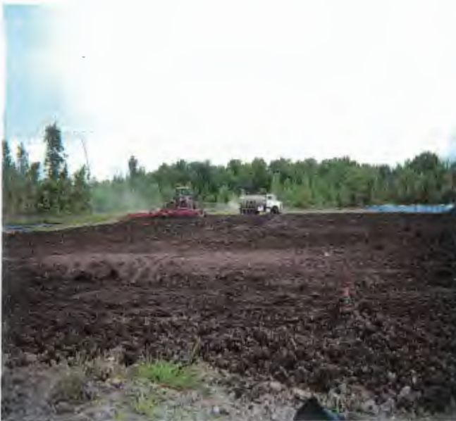
Spreading and mixing Stabilized Soil
