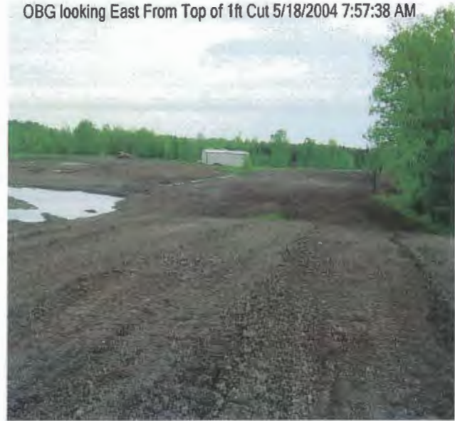
OBG Looking East From 1 ft. Cut at Grid K5
