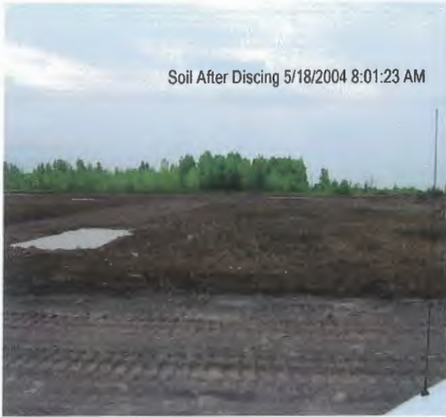
Soil After Discing
