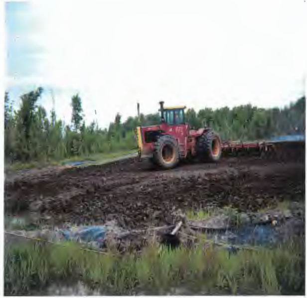
Mixing Soil During Soil Stabilization
