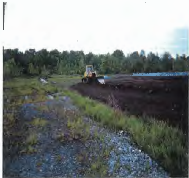
Removing Stabilized Soil in 1' Lifts
