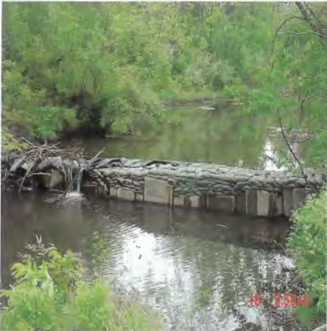
Reeder Creek South Dam
