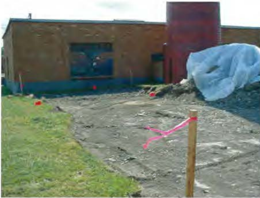
Photograph #3 - Top six inches of clean soil was excavated and staged on site for future backfill at SEAD 39.
