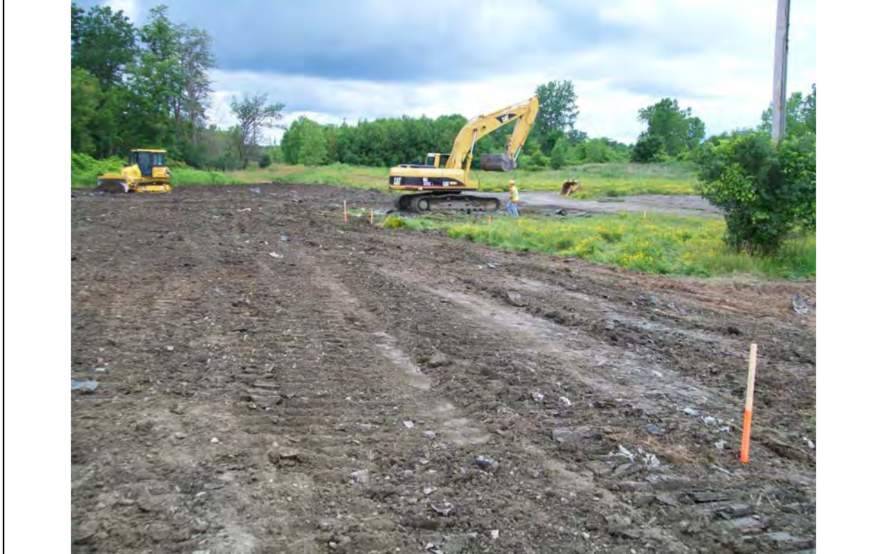
Photo: 12 Date: 7/8/2009 Site: SEAD-5 Description: Excavator running North-South across surface to compact of SEAD-59/71 stockpile soil cap.
