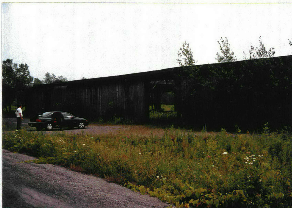
PHOTO # 34 TYPICAL STORAGE SHED
