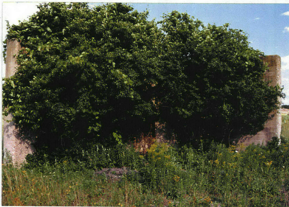
PHOTO # 40 EXPLOSIVE SCRAP FURNACE
