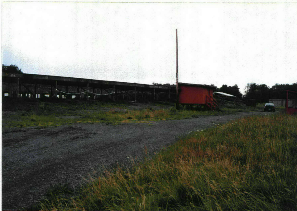
PHOTO # 28 SMALL ARMS RANGE NEAR AIRFIELD
