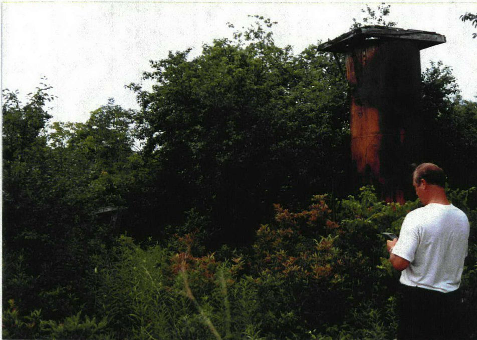
PHOTO # 31 TOWER AND SHACK AT SMALL ARMS RANGE NEAR THE LAKE HOUSING AREA
