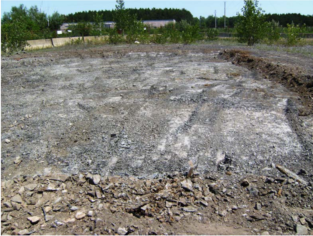
Two-Foot Excavation Looking North
