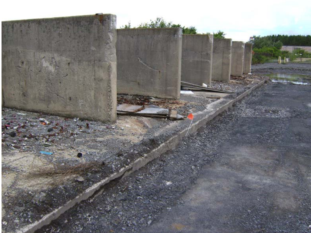
SEAD-121C Initial Excavation (1-foot) in Vicinity of Well MW121C-3 Looking North-Northeast
