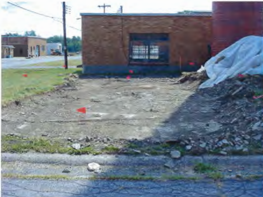
Photograph #2– View of the excavation area and post-excavation sample locations, marked with red flags at SEAD 39.
