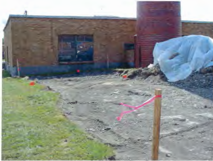
Photograph #3 - Top six inches of clean soil was excavated and staged on site for future backfill at SEAD 39.
