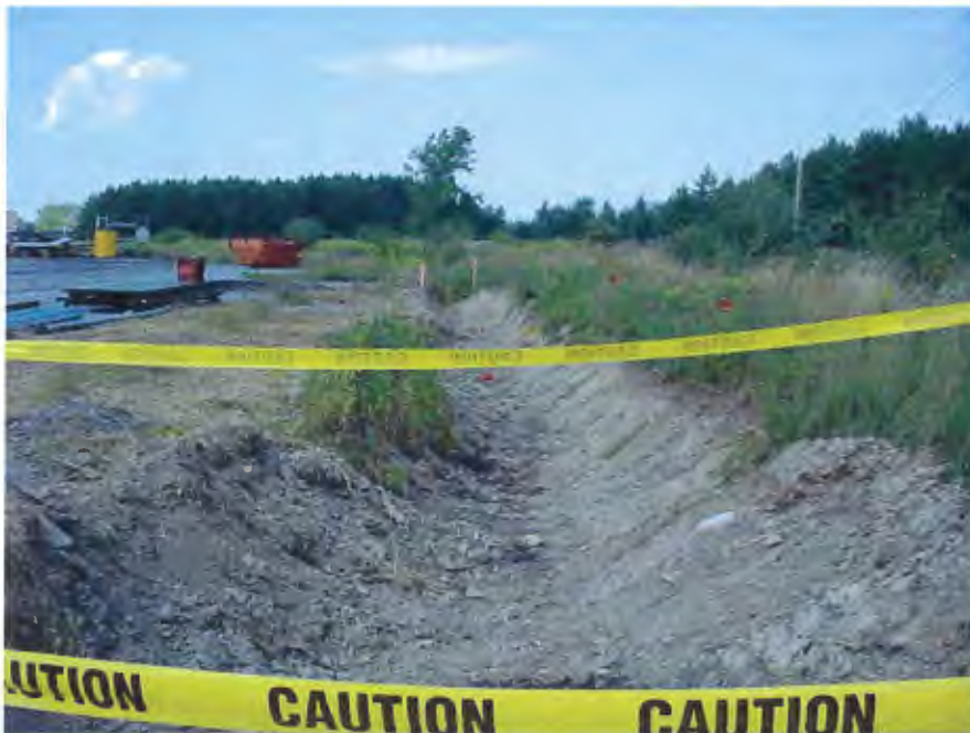
Photograph #6 – Caution tape was set up around the ditch with 6-ft excavation at SEAD 40.
