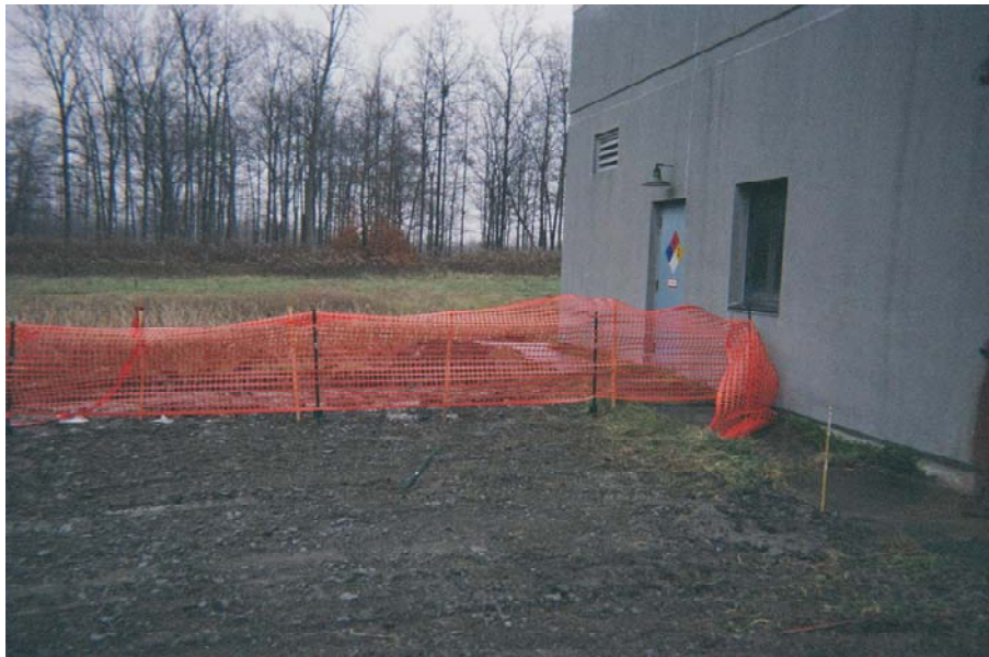
Looking East towards excavation – snow fence to help prevent injury
