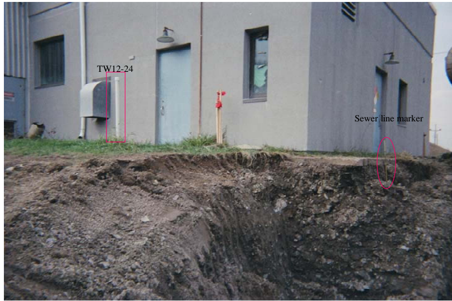
Horizontal view of previous excavation photo
