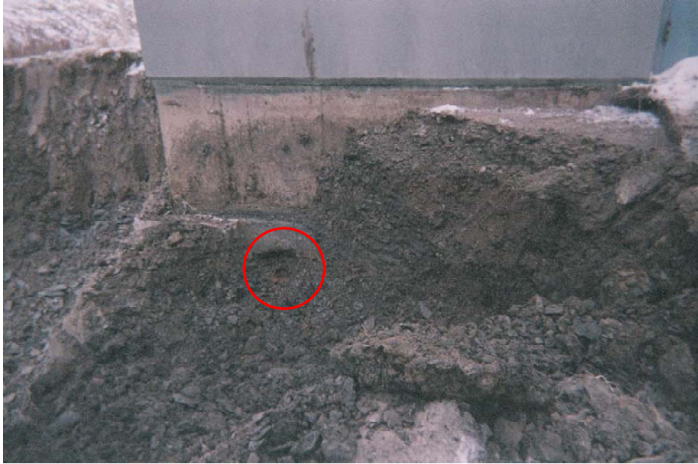
Location of 4-inch Ductile Iron pipe exiting Building 813 foundation
