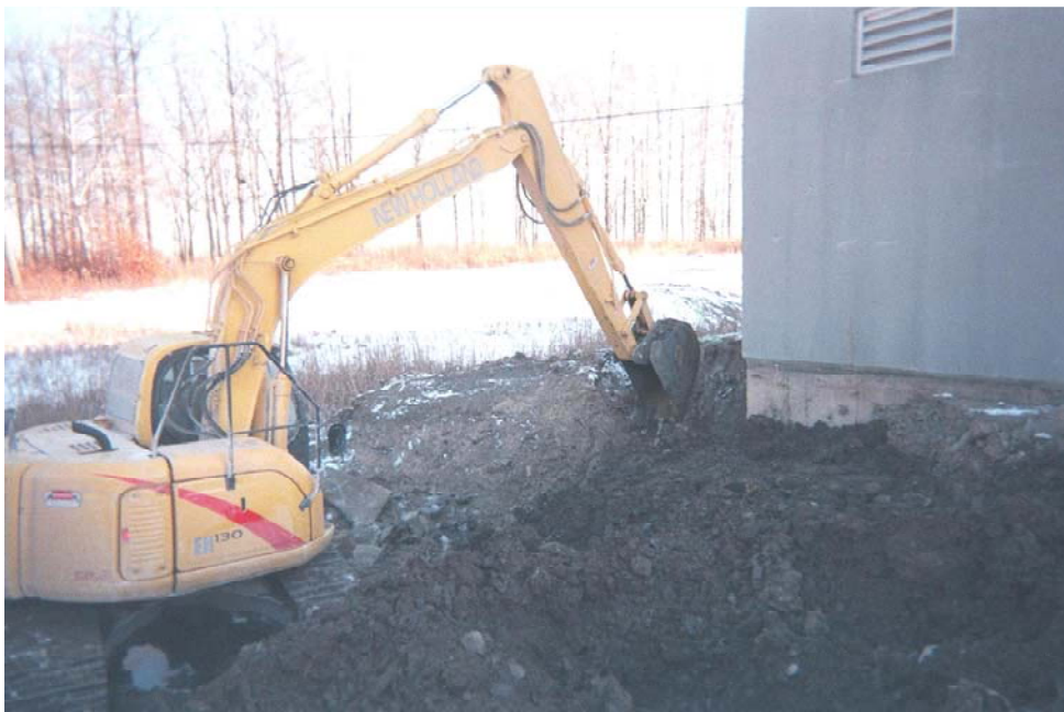
Phase III excavation near NE corner of Building 813
