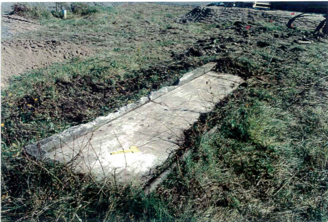
FIGURE 21 - Structure 1 (view to ESE)
