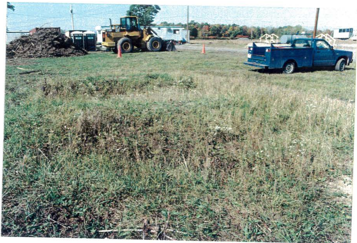
FIGURE 26 - Structure 3 with staging area rear (view to NW)
