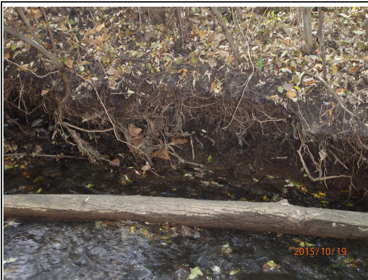
Photo #33 – Looking west at the Reeder Creek embankment on the side of the OB Grounds. Visible soil within embankment shows signs of scouring. The roots from vegetation are helping keep embankment soils in place.
