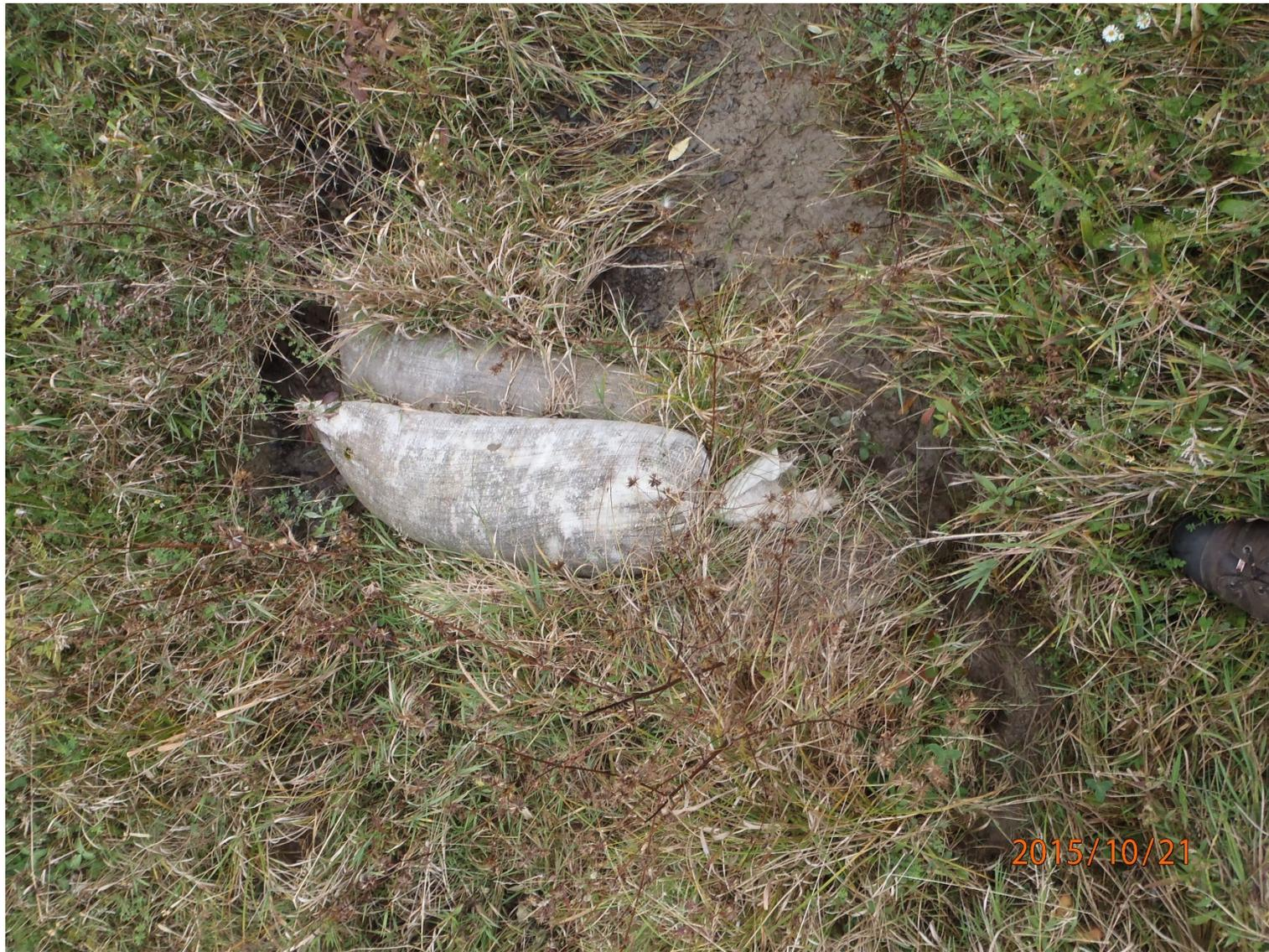
Photo #37 – View of sand bags in drainage ditch that leads down to Reeder Creek, located between MW23-1 and MW23-2. Flow through the drainage ditch during strong rain events has caused minor erosion around the perimeter of the sandbags. Erosion has created a new preferential flow path around the sand bags.
