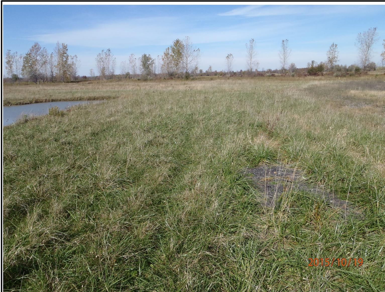
Photo #08 – Grid I6. Crushed shale used to fill and grade tire ruts in 2014 is still in place. No erosion or disturbances to the cap were observed. The grid is well vegetated. View to the north.
