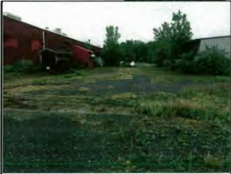
Status as of: 6/1/15 Photo ID: IMG_6566.JPG Description: SEAD-121C
