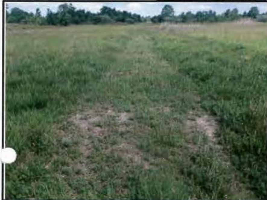
Status as of: 6/2/15 Photo ID: P604004.JPG Description: View of Biowall C.
