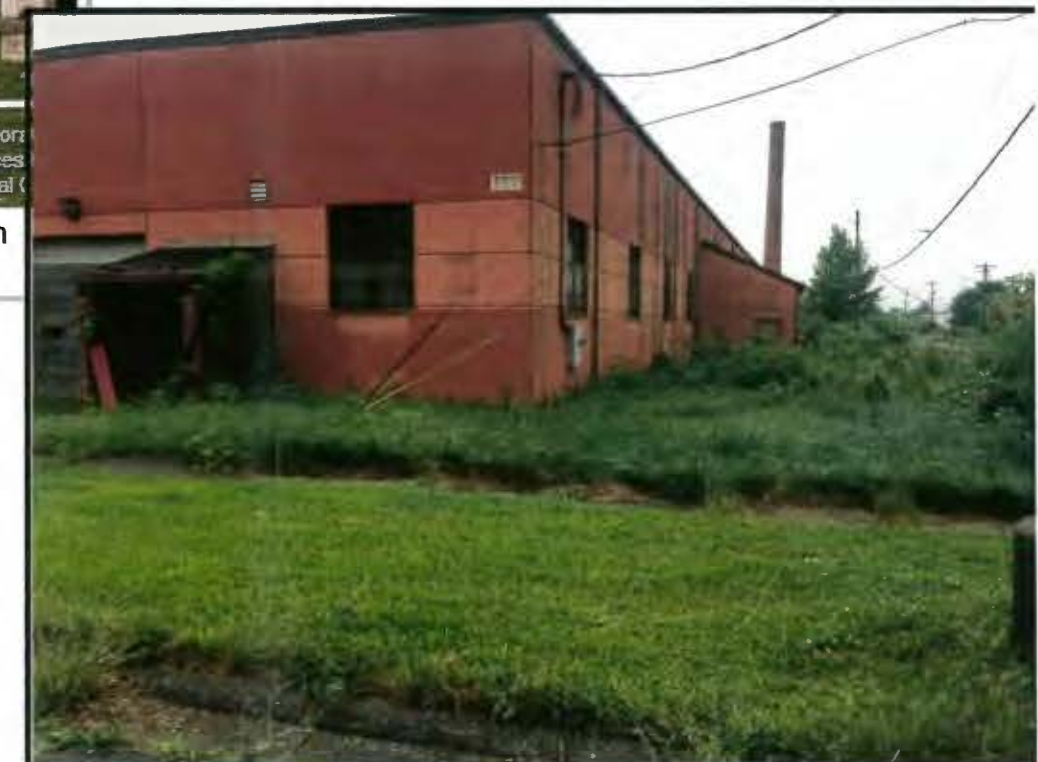
Status as of: 6/1/15 Photo ID: img_6540.JPG Description: SEAD-39, area of blowdown leaching pit.
