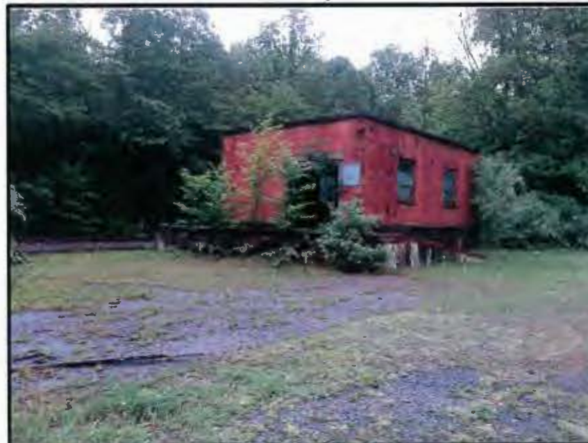
Status as of: 6/1/15 Description: Building 307
