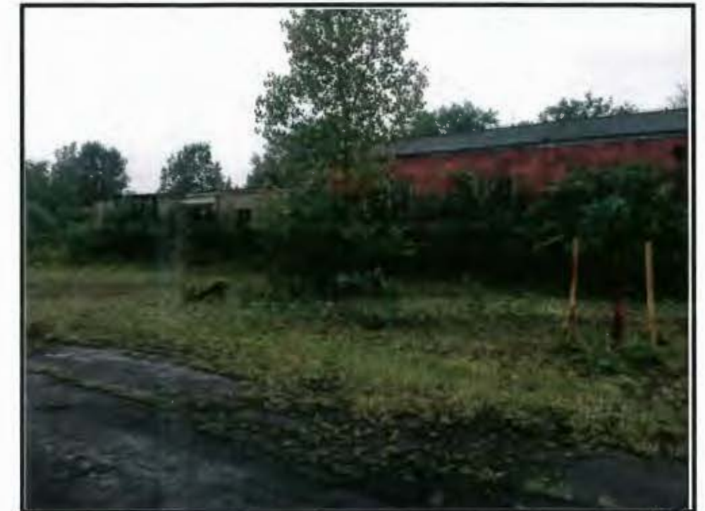
Status as of: 6/1/15 Description: SEAD-66
