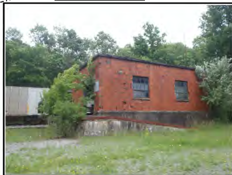
Status as of: 6/26/2017 Description: Building 301
