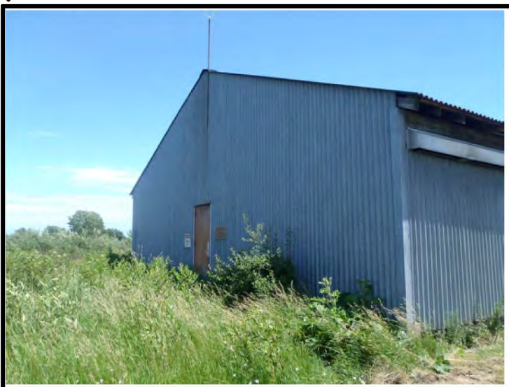
Status as of: 6/26/2017 Description: Building 307 Photo ID: P6260033.JPG
