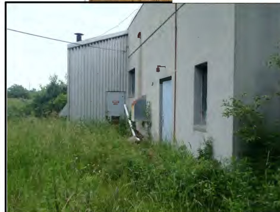
Status as of: 6/26/2017 Photo ID: P6130024.JPG Description: SEAD-12
