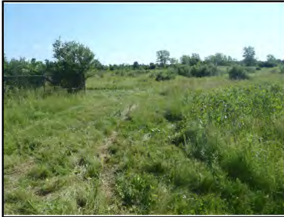
Status as of: 6/26/17 Photo ID: P6280089.JPG Description: Looking north across portion of biowall within the Ash Landfill.
