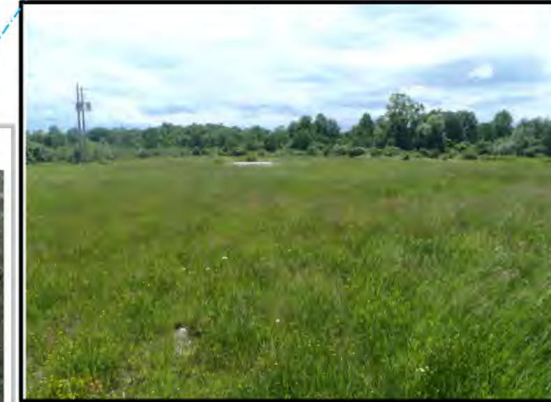
Status as of: 6/26/2017 Photo ID: P6260058.JPG Description: SEAD-17, Building 367 foundation.
