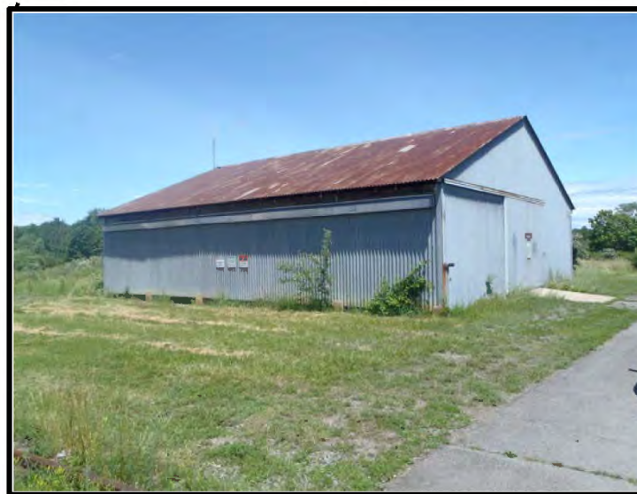
Status as of: 6/26/2017 Description: Building 307 Photo ID: P6260032.JPG
