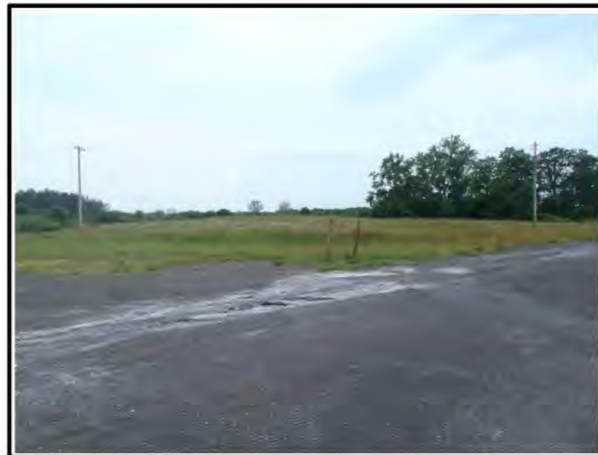
Status as of: 6/29/2017 Description: SEAD-5 cap Photo ID: P6290148.JPG
