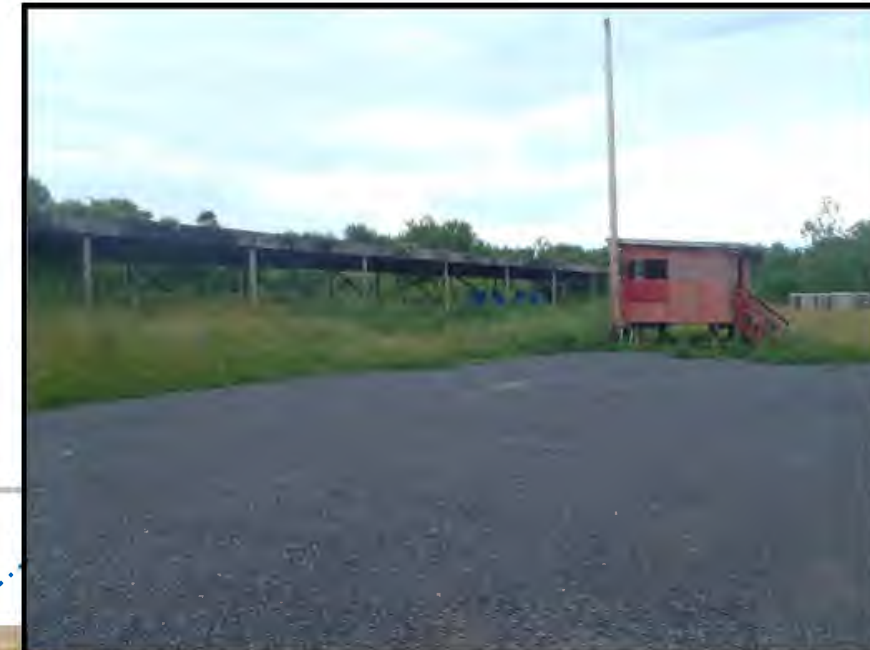
Status as of: 6/26/2017 Description: SEAD-122B Photo ID: P6260074.JPG
