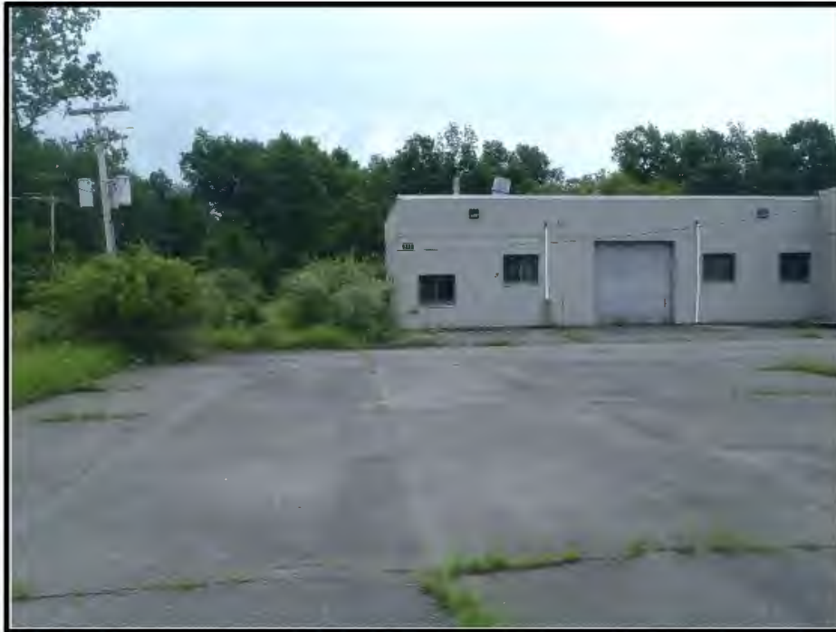
Status as of: 6/26/2017 Photo ID: P6290142.JPG Description: SEAD-12
