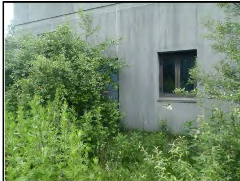
Status as of: 6/26/2017 Photo ID: P6290143.JPG Description: SEAD-12
