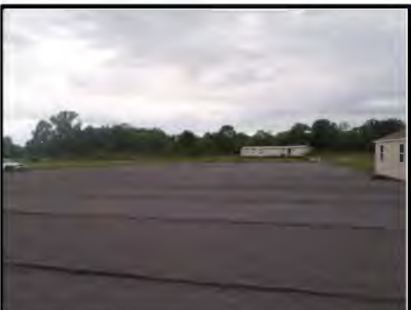
Status as of: 6/26/2017 Photo ID: P6260077.JPG Description: SEAD-122E
