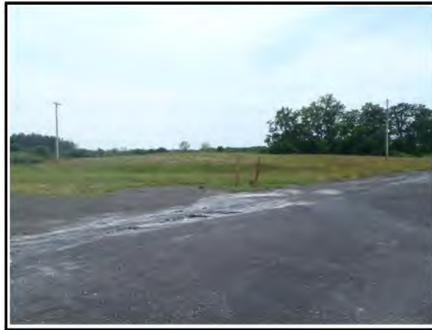
Status as of: 6/29/2017 Description: SEAD-5 Cap Photo ID: IMG_3599.JPG
