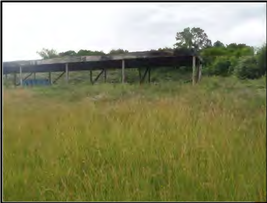
Status as of: 6/26/2017 Description: SEAD-122B Photo ID: P6260073.JPG
