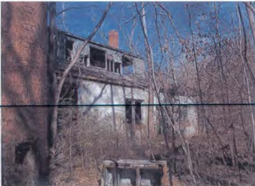
Photograph 2: Incinerator Building – Back
