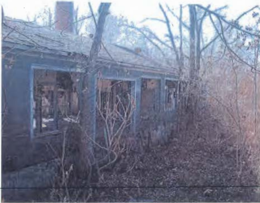
Photograph 1: Incinerator Building – Front
