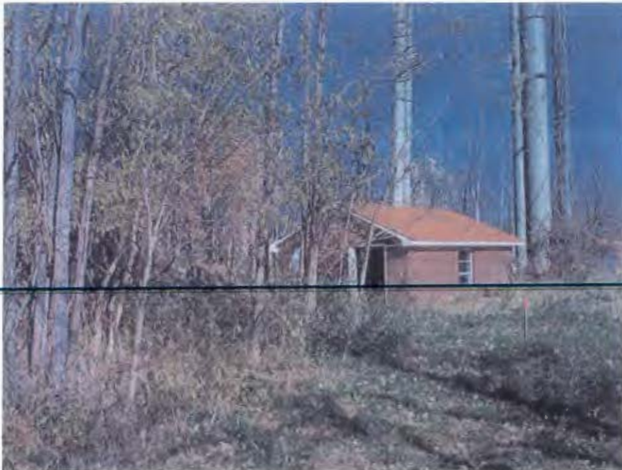
Photograph 6: Water Tower and Water Building
