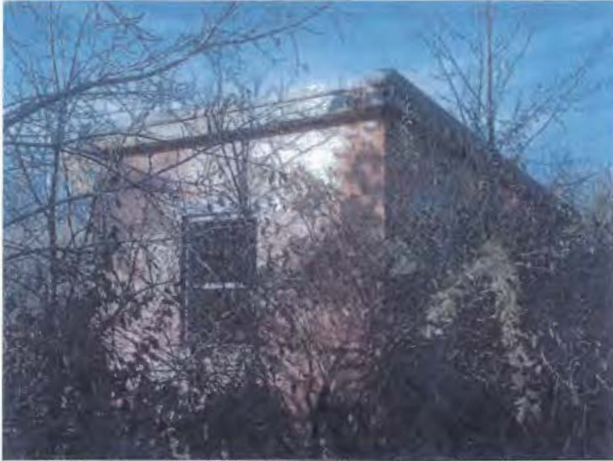
Photograph 5: Waste Water Treatment Plant – Screen Control Building
