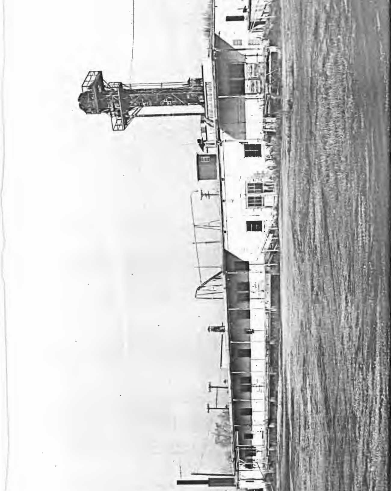
Illustration 15 "Popping" Plant (Building 311). Seneca's "popping" plant, built in 1943, was one of five such plants in operation in the United States during World War II. Cleaned ammunition shells were conveyed through the cooling tower at the south end of the building before being dropped into rail cars. (Source: Field inventory photograph, 1983, Barbara Hightower, Building Technology, Inc.)
