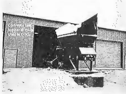
14. Conveyor hopper for metal to be Separated
