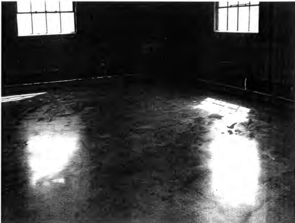
After completion of rinsing operations.
