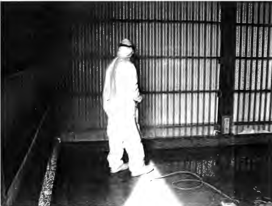
Washing inside of Bldg 307.
