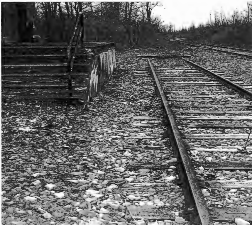
Location of railroad bed adjacent to building.
