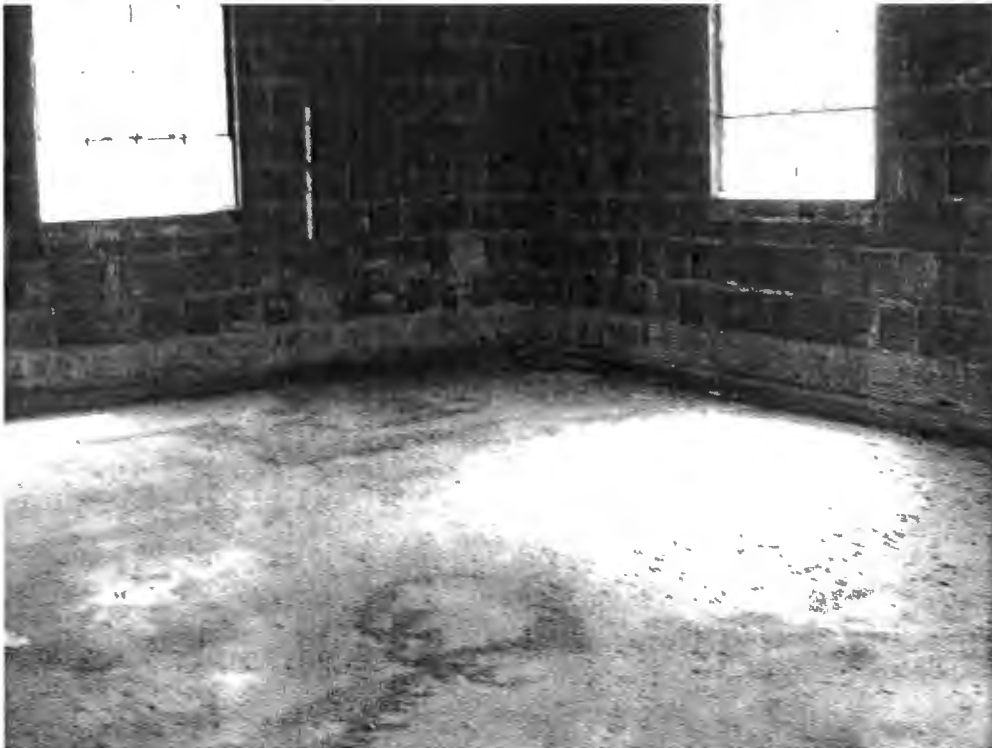
Building 301 after debris removal.
