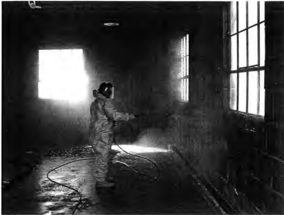
Performing cleaning operations at Bldg 301.
