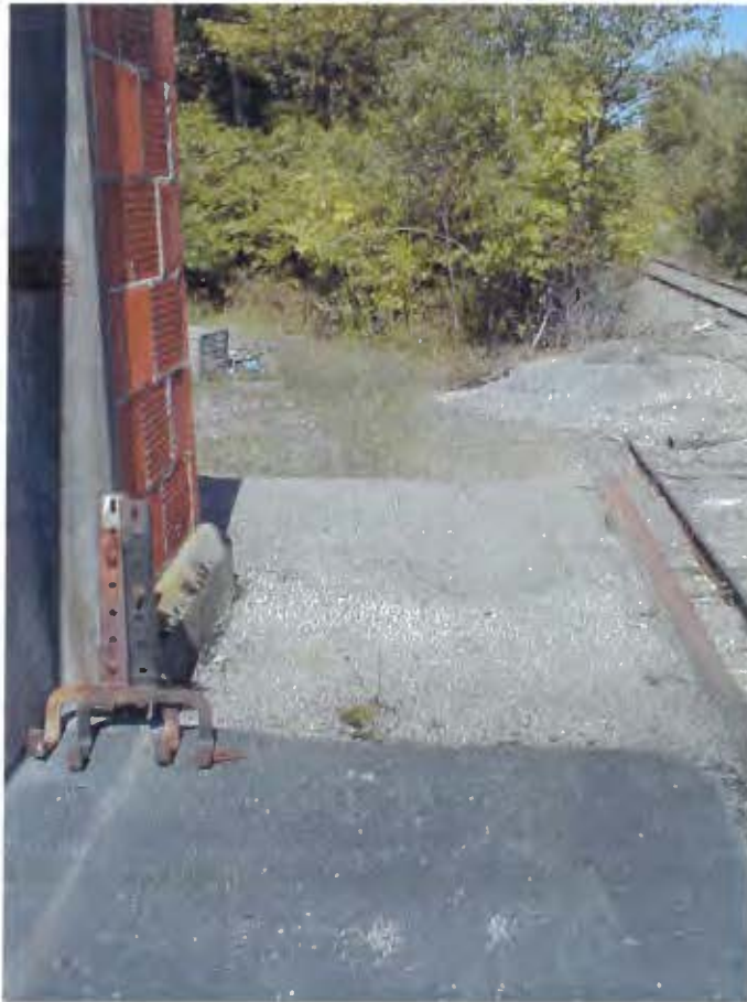
Figure 4: Northeast corner of Building 301 (SEAD-2) Loading Dock with Asphalt/Gravel Traction covering
