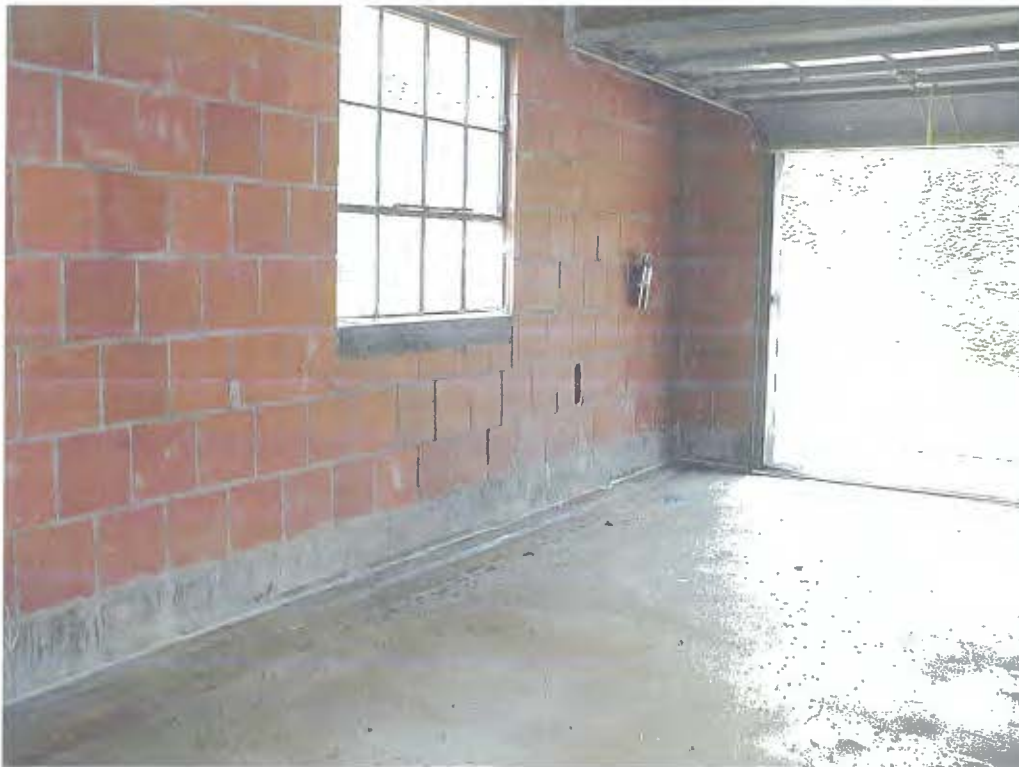
Figure 2: Interior of Building 301 (SEAD-2) looking north prior to decontamination
