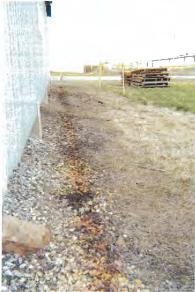
Figure 6: Exterior of Building 307 facing south
