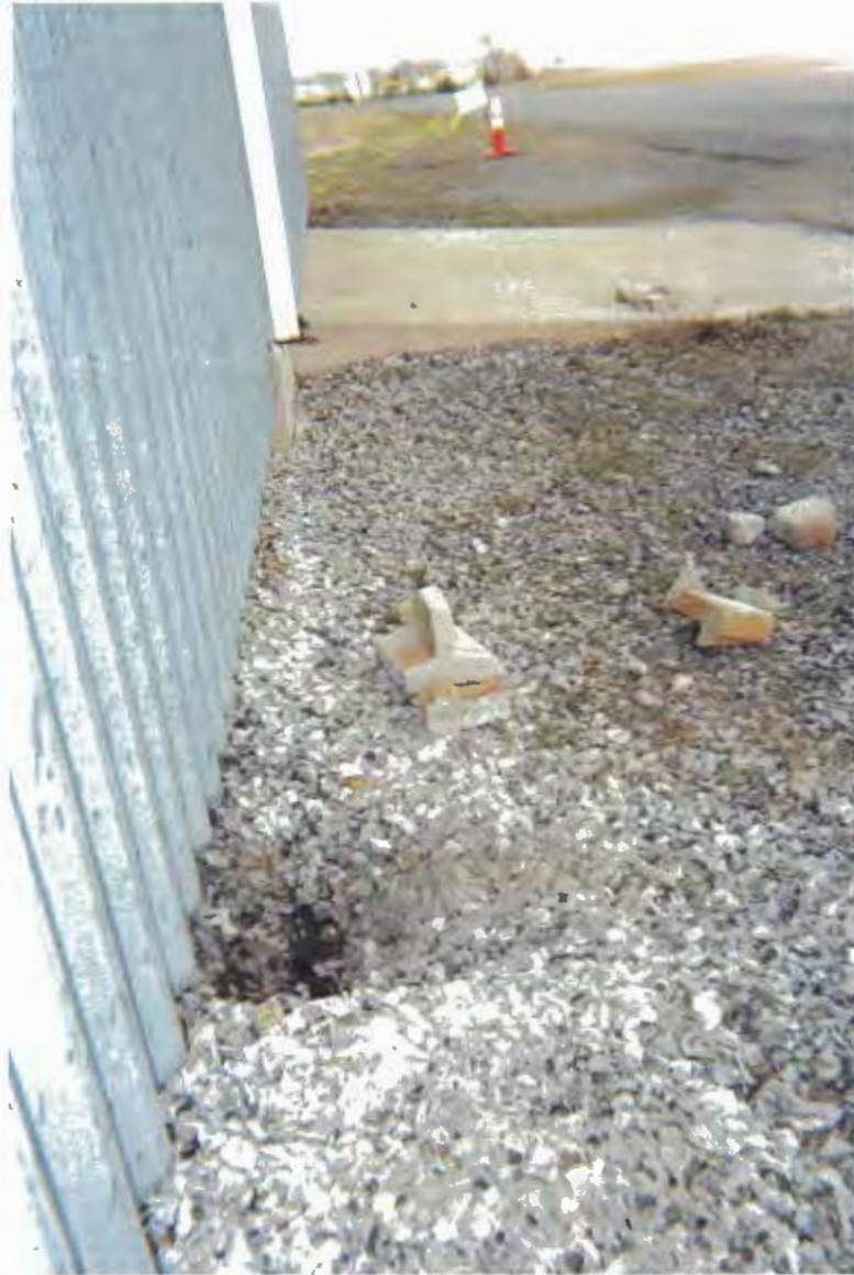
Figure 7: Southern exterior end of Building 307 (SEAD-1) facing West.
