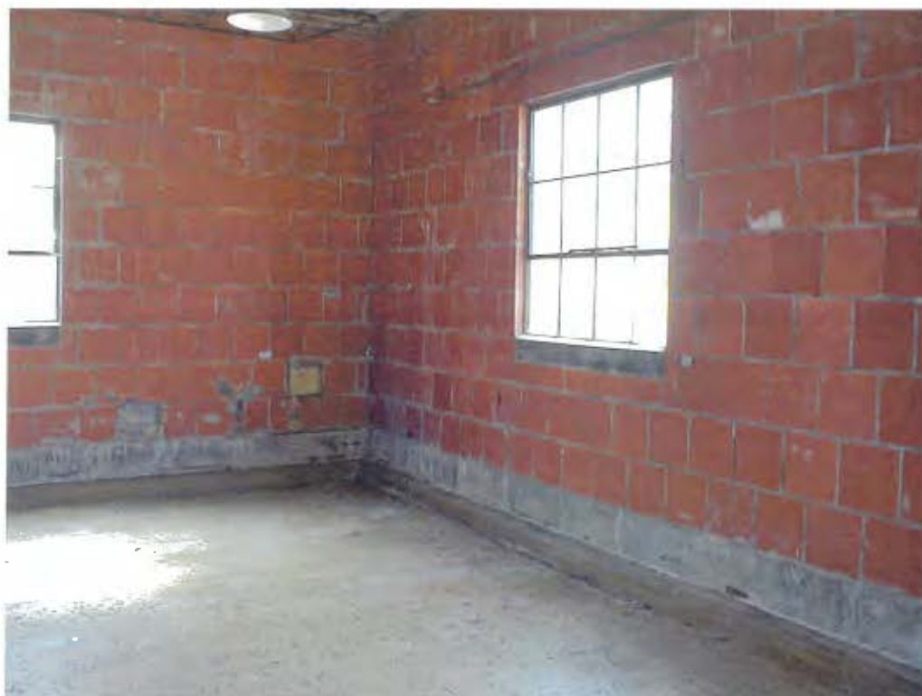
Figure 3: Interior of Building 301 (SEAD-2) looking southwest prior to decontamination
