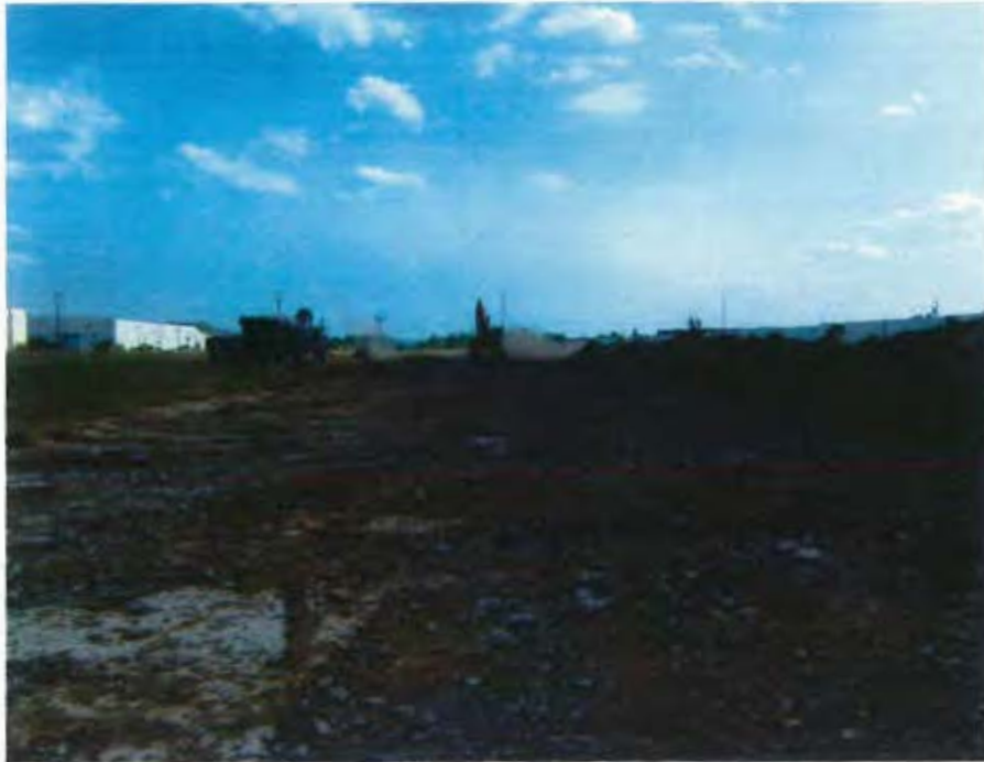
SEAD-1211 Former Ore Pile Location 2 During Soil Load Out Looking South
