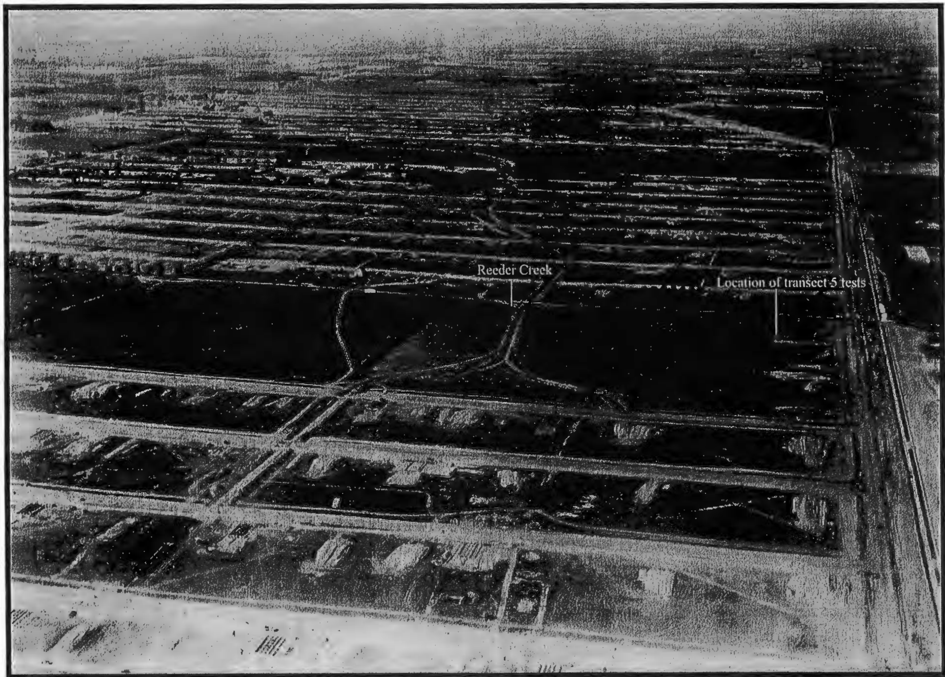
Figure 10. Aerial photograph of SEDA, September 1941, view to north showing igloo construction (from SEDA archives).
