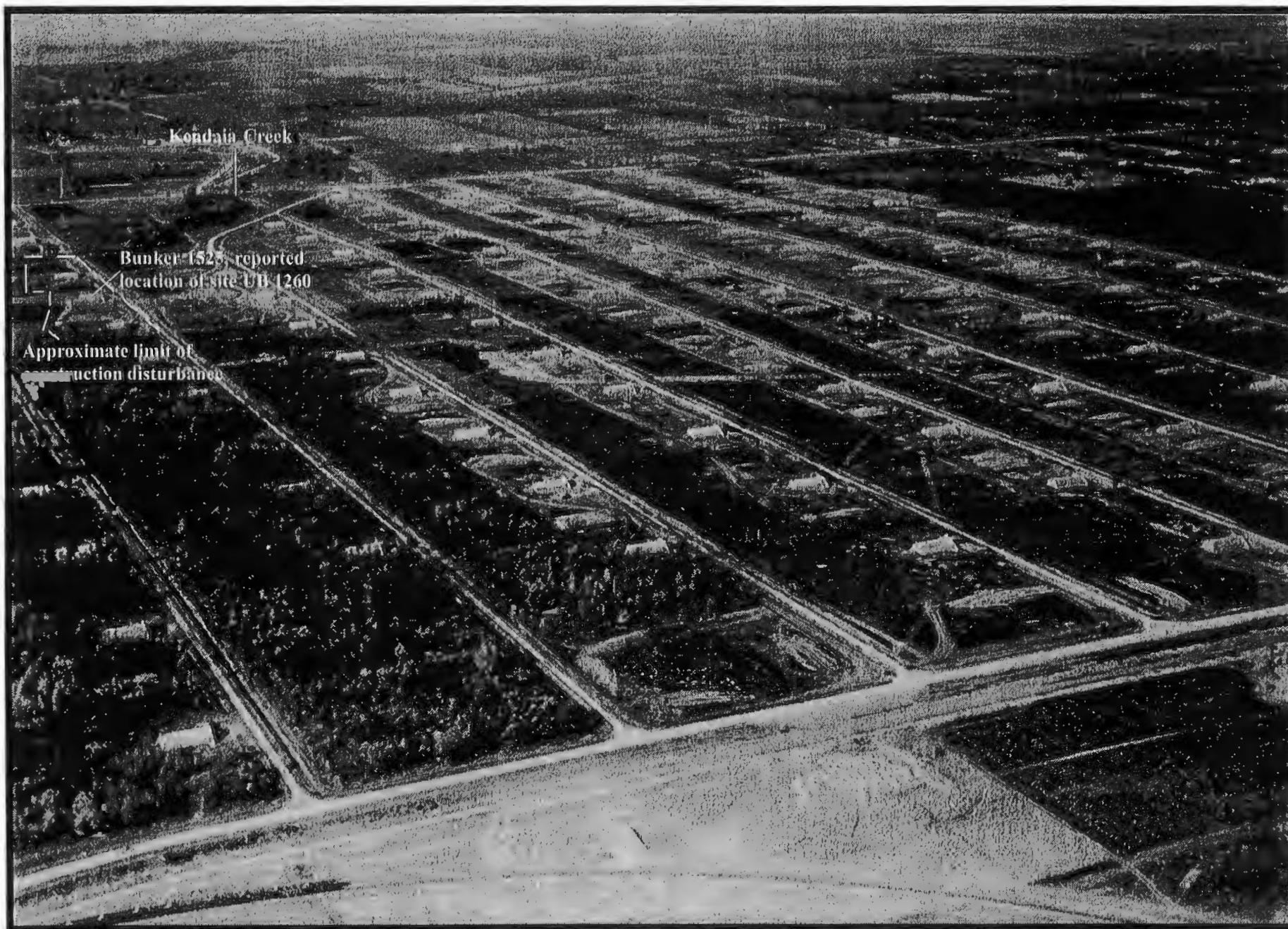
Figure 8. Aerial photograph of SEDA, October 1941, view to northwest, showing igloo construction (from SEDA archives).
