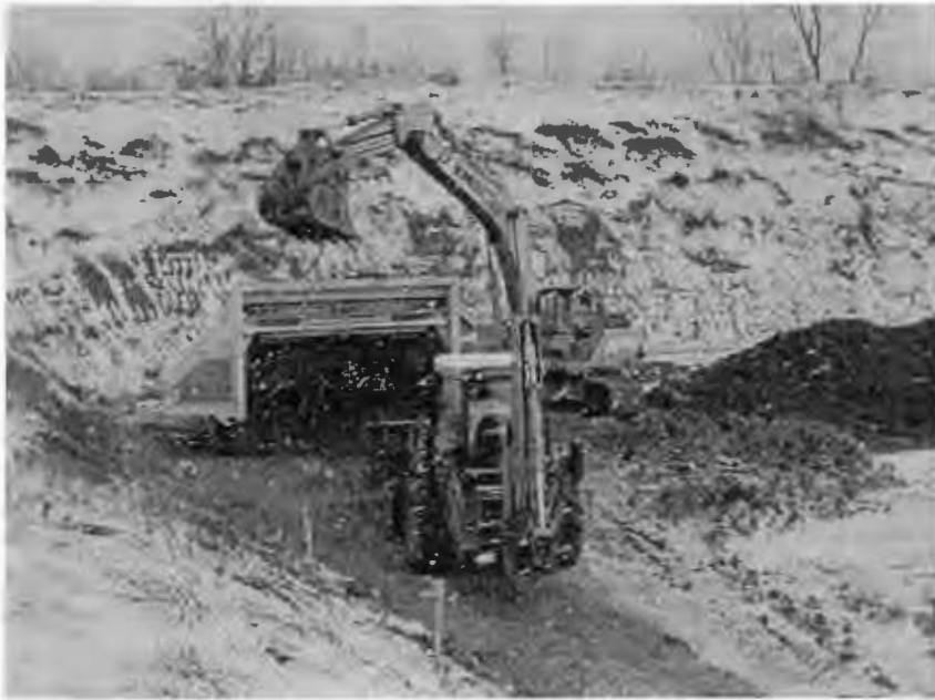
Screening excavated soils.
