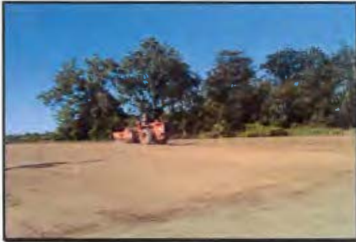
10-ton vibratory roller compacting the final engineered cover surface
