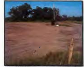
Completed engineered cover at SEAD-5
