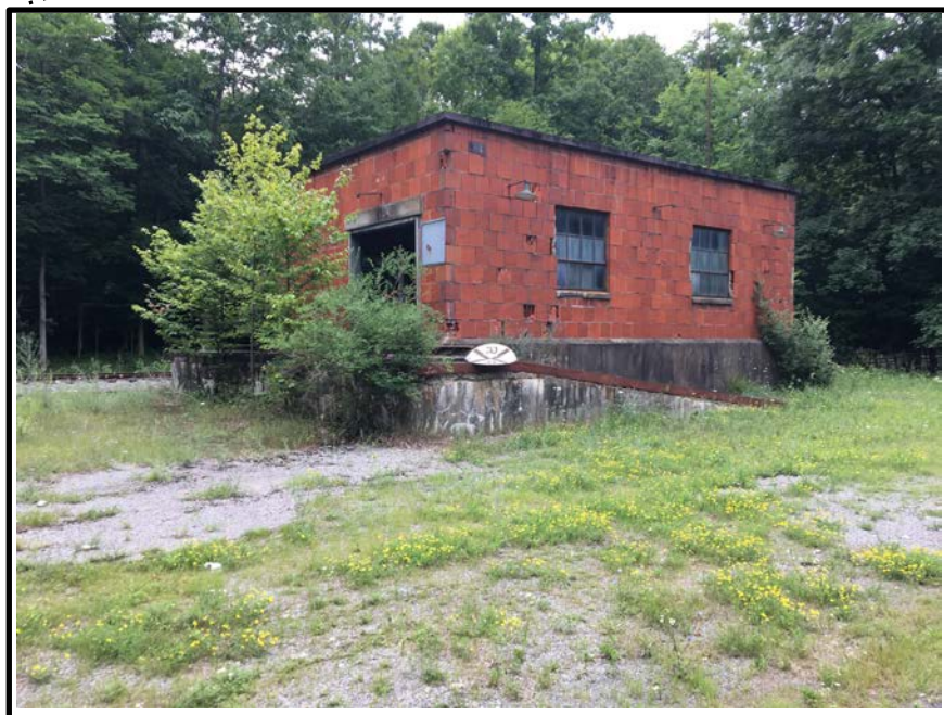
Status as of: 7/22/2020 Description: Building 301
