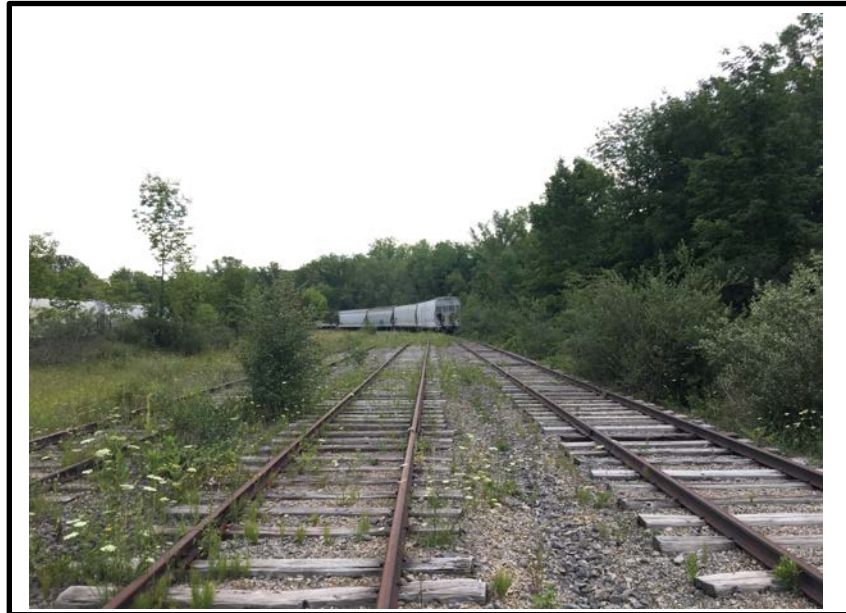
Status as of: 7/22/2020 Photo ID: IMG_3913.jpg Description: SEAD-64B
