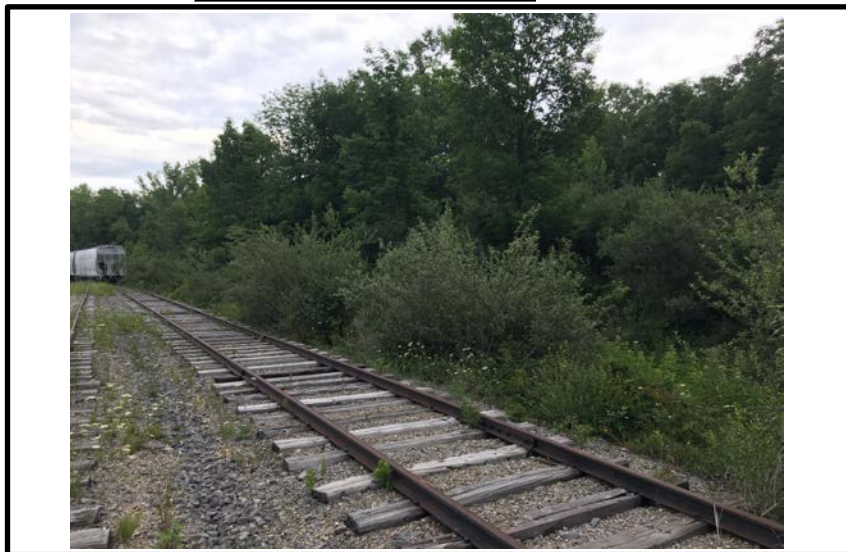
Status as of: 7/22/2020 Photo ID: IMG_3912.jpg Description: SEAD-64B
