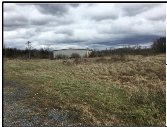
Status as of: 11/22/2019 Grid P10. No erosion or disturbances to the cap were observed. The grid is well vegetated. Wet swampy area in northeast portion of grid. View to the southeast
