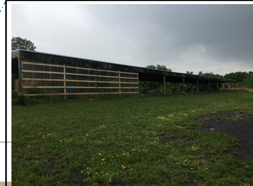
Status as of: 7/22/2020 Photo ID: IMG_3939.JPG Description: SEAD-122B
