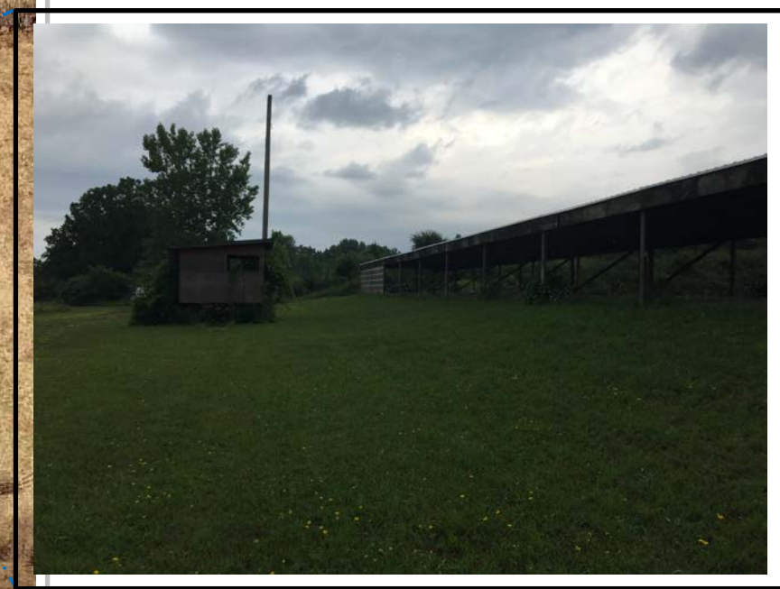
Status as of: 7/22/2020 Photo ID: IMG_3944.JPG Description: SEAD-122B
