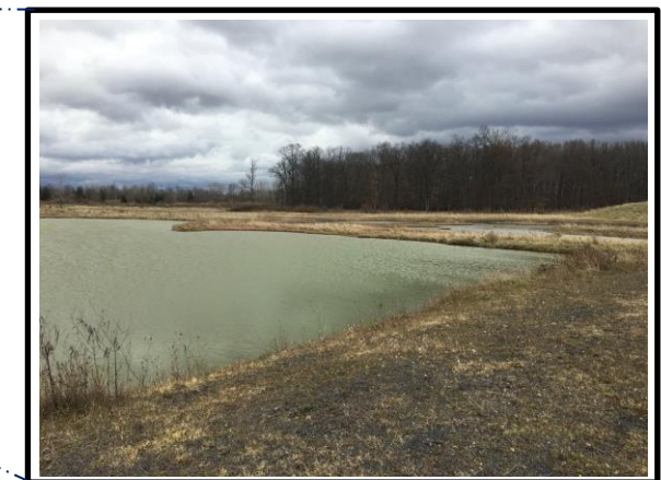
Status as of: 11/22/2019 Grid L9. The grid is well vegetated along the edges of the pond; thin areas noted in center of grid and along slopes. View to the southeast
