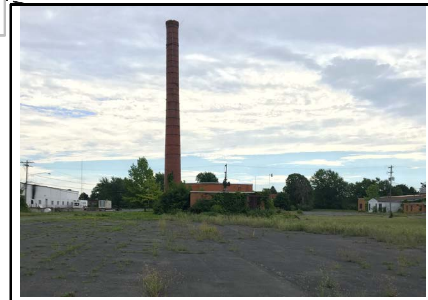
Status as of: 7/22/2020 Photo ID: IMG_3873.jpg Description: SEAD-39, area of blowdown leaching pit.
